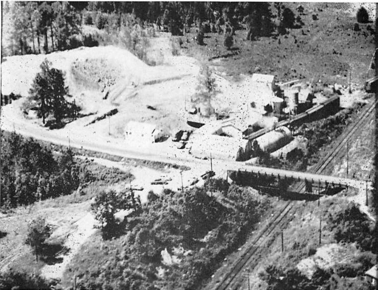
Figure 10.—American Colloid Company's plant at Aberdeen, Monroe County. NW  $\frac{1}{4}$ , NW  $\frac{1}{4}$ , SW  $\frac{1}{4}$ , Sec. 2, T. 15 S., R. 7 E. Plant processes Eutaw bentonite for use as foundry bonding clay. Photo by American Colloid Company.
