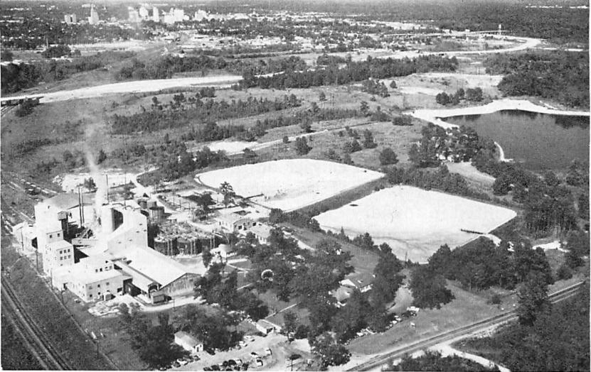
Figure 9.—Filtr Corporation's bentonite activation plant at Jackson, Hinds County. Plant processes Mississippi and out-of-state clay for absorbent and other uses. Photo by Manley, Tucson.
