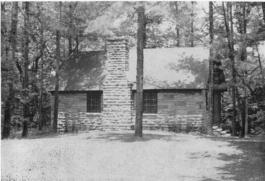
Figure 31.—Cabin constructed of Highland Church sandstone in Tishomingo State Park, Tishomingo County. (M.G.S. Bull. 86, Fig. 27).
