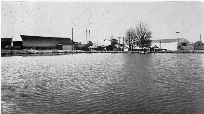
Figure 12.—Wyandotte Chemical Corporation plant located at Blue Mountain, Tippah County. Plant produces a fired clay aggregate from the Porters Creek formation used for absorbent purposes. Photo by Wyandotte.
