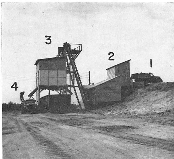
Figure 4.—Mississippi State Department of Agriculture agricultural lime plant near Cedar Bluff, Clay County. (1) unloading raw material, (2) crusher shed, (3) storage and loading bin, (4) rail and highway transportation. (M.G.S. Bull. 86 Fig. 33).
