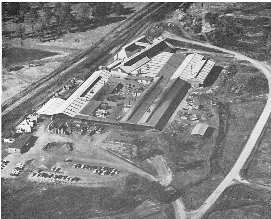
Figure 15.—Tri-State Brick & Tile Company Plant near Jackson: (1) pit opened in clay loam, (2) dry clay storage, (3) clay preparation facilities, (4) driers and tunnel kilns, (5) finished bricks, (6) rail and truck loading areas. Photo by Hand Portraits, December 1963.
