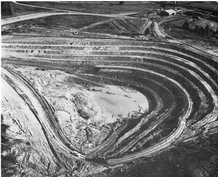
Figure 17.—Open-cut pit of the Lightweight Aggregate Division, Jackson Ready-Mix Concrete (NE.  $\frac{1}{4}$ , NW.  $\frac{1}{4}$ , Sec. 36, T. 7 N., R. 1 W.). The mine is over 60 feet deep. Note the several tiered benches from which the clay is worked.—Bob Hand photo.
