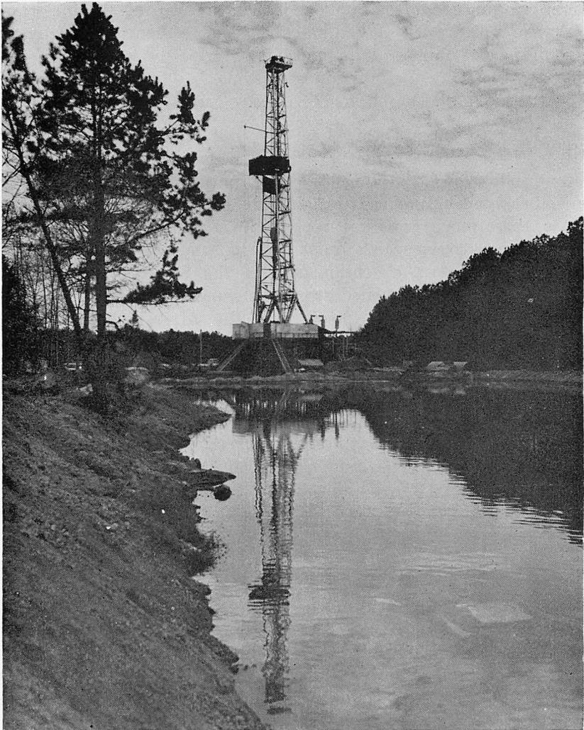
Figure 33.—Shell Oil Company No. 1 Garrett, Sec. 28, T. 4 N., R. 3 E., Rankin County. Potential high sulfide gas discovery from Smackover formation at a depth of approximately 20,000 feet. Photo by Shell Oil Company, 1969.
