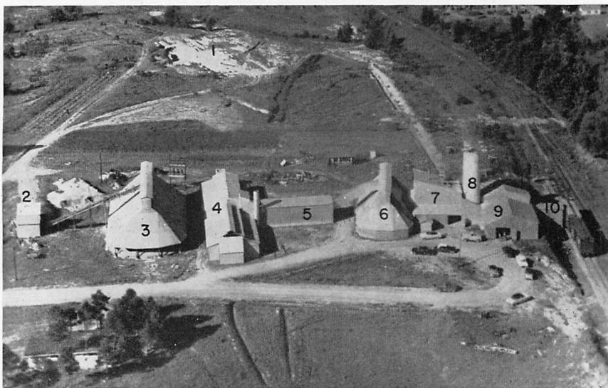
Figure 13.—Oil-Dri Corporation plant located in Ripley, Tippah County. Products include a fired clay aggregate used for absorbent and deodorizing purposes: (1) clay pit in Porters Creek formation, (2) shredding shed, (3) drying shed, (4) kiln building, (5) cooler, (6) storage shed, (7) crushing and sizing, (8) silos, (9) packaging, and (10) loading. Photo by Richard Allin.
