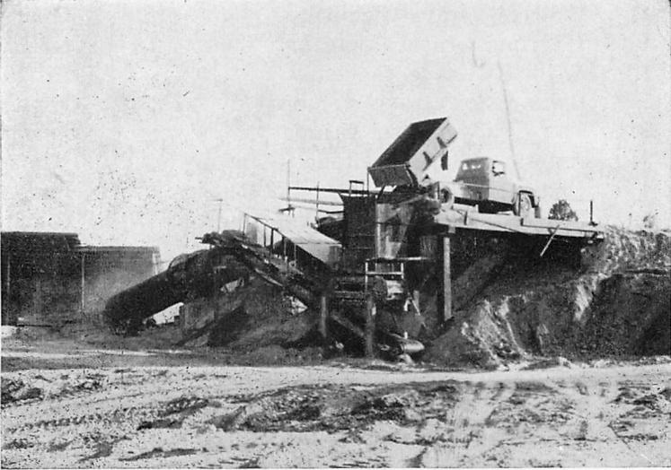
Figure 21.—Tri-State Sand Company's plant located in Tishomingo County. Plant produces foundry sand from the Eutaw formation. (M.G.S. Bull. 86, Fig. 14).
