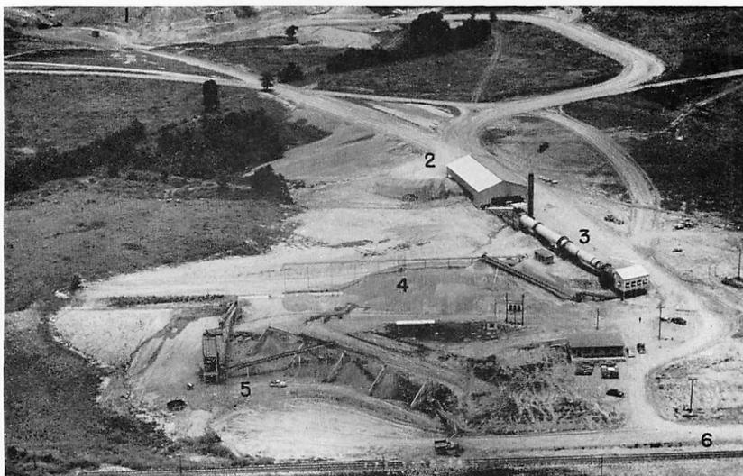
Figure 16.—Lightweight Aggregate Division plant of Jackson Ready-Mix Concrete at Cynthia: (1) pits opened in the Yazoo clay, (2) Clay dry shed, (3) rotary kiln, (4) cinder storage area, (5) grinding, screening and storage of graded aggregates, and (6) rail or truck shipping facilities. (M.G.S. Bull. 86, Fig. 24).—Frank Noone photo, July 2, 1958.
