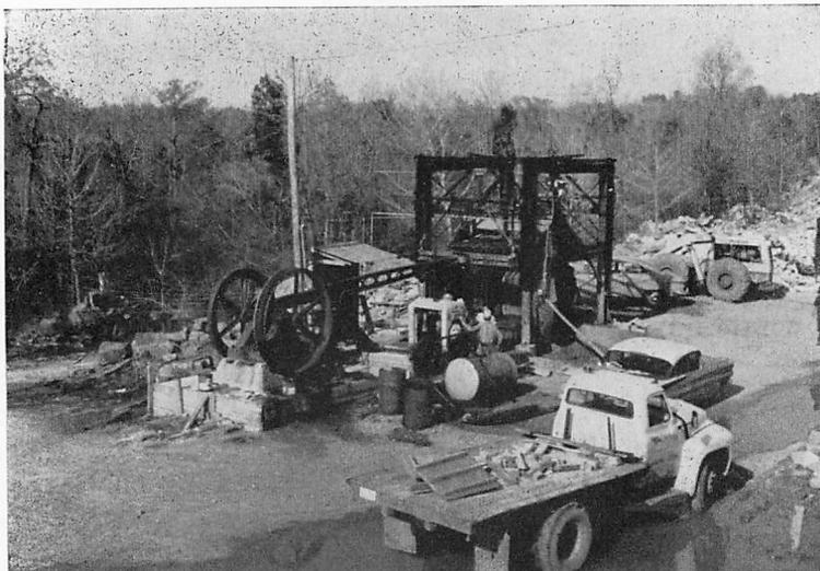
Figure 32.—Gang mill quarry of Mississippi Stone Company located in NW  $\frac{1}{4}$ , NE  $\frac{1}{4}$ , Sec. 7, T. 6 S., R. 11 E., Tishomingo County. Company produces standard grades of dimension stone. (M.G.S. Bull. 86, Fig. 28).
