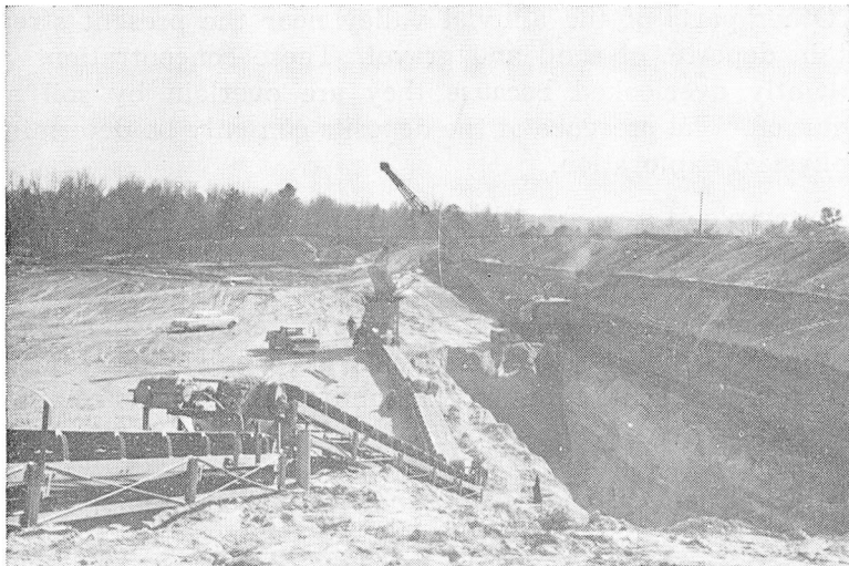
Figure 23.—Excavating sand and gravel by dragline. Conveyor transports material to classifier screen. Location at gravel pit in SW \frac{1}{4} , NW \frac{1}{4} , sec. 31, T. 2 N., R. 1 W. March 1968.
