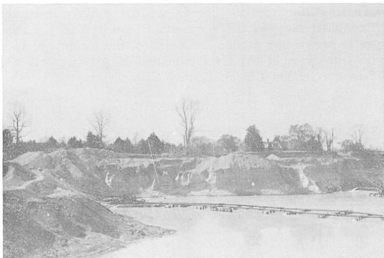
Figure 22.—Excavating sand and gravel by hydraulic dredge. Material is transported to classifier screens by pipeline. Location at gravel pit in SE \frac{1}{4} , SE \frac{1}{4} . sec. 31, T. 2 N., R. 1 W. March 1968.
