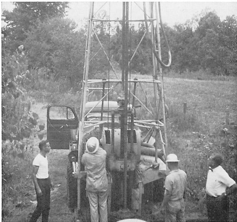
Figure 1.—Survey's Failing 750 rotary drilling rig being used in coring the type locality of the Yazoo clay (M.G.S. Bull. 100, Fig. 31). Norman A. Mott photo. September 27, 1963.
