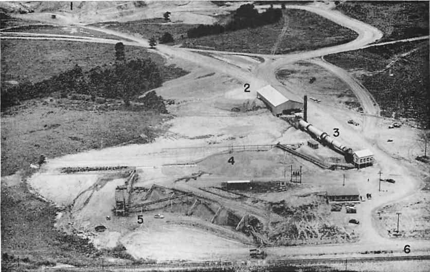
Figure 14.—“Miss-Lite” aggregate plant of Jackson Ready-Mix Concrete at Cynthia, Hinds County: (1) pits opened in the Yazoo clay, (2) clay dry shed, (3) rotary kiln, (4) cinder storage area, (5) grinding, screening and storage of graded aggregates, and (6) rail or truck shipping facilities. (M.G.S. Bull. 86, Fig. 24).—Frank Noone photo, July 2, 1958.
