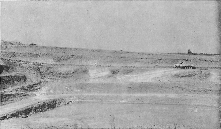
Figure 15.—Open-cut pit of Jackson Ready-Mix Concrete at Cynthia, Hinds County (SE.  $\frac{1}{4}$ , SW.  $\frac{1}{4}$ , Sec. 25 and NE.  $\frac{1}{4}$ , NW.  $\frac{1}{4}$ , Sec. 36, T.7 N., R.1 W.). The mine is over 60 feet deep and has several tiered benches from which the clay is worked. (M.G.S. Bull. 88, Fig. 9). September 4, 1959.
