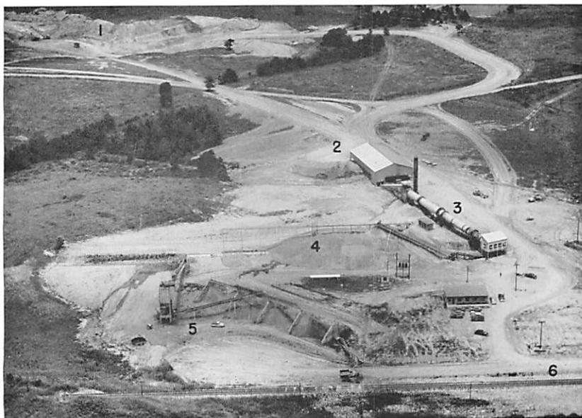
Figure 24.—“Miss-Lite” aggregate plant of Jackson Ready-Mix Concrete at Cynthia, Hinds County: (1) pits opened in the Yazoo clay, (2) clay dry shed, (3) rotary kiln, (4) cinder storage area, (5) grinding, screening and storage of graded aggregates, and (6) rail or truck shipping facilities. (M.G.S. Bull. 86, Fig. 24). Frank Noone photo, July 2, 1958.
