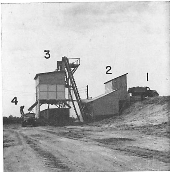
Figure 21.—Plant of Division of Lime, Mississippi Department of Agriculture, Clay County: (1) truck unloading chalk lumps, (2) crusher shed, (3) storage and loading bin, (4) rail and highway transportation. Division of Lime photo, December, 1958. (M.G.S. Bull. 86, Fig. 33).
