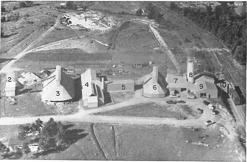
Figure 26.—Plant of Howell-Southern Products, Inc., Ripley, Tippah County, which produces fired clay aggregate for absorbent and deodorizing purposes: (1) clay pit—basal Porters Creek, (2) shredding shed, (3) dry shed, (4) kiln building, (5) cooler, (6) product storage, (7) screening and crushing, (8) silos, (9) bagging, and (10) loading. Looking south. (M.G.S. Bull. 86, Fig. 22). Richard Allin photo, December, 1958.
