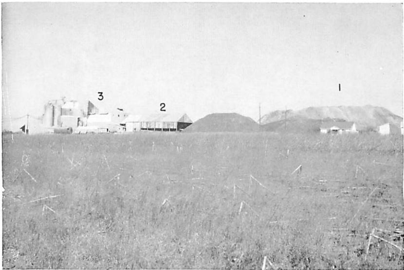
Figure 23.—"Dixie Bond" plant of Eastern Clay Products Department of International Mineral & Chemical Corporation at Smithville, Monroe County: (1) stock pile, approximately 65,000 tons of bentonite, (2) dry shed, (3) kiln, mill and storage housing. (M.G.S. Bull. 86, Fig. 19). Eastern Clay Products photo, January 21, 1959.
