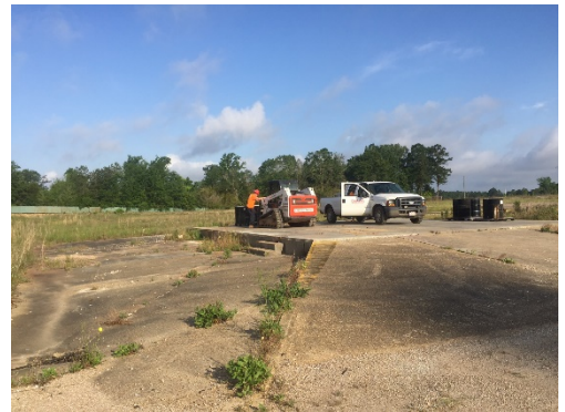
Relocating IDW Drums
