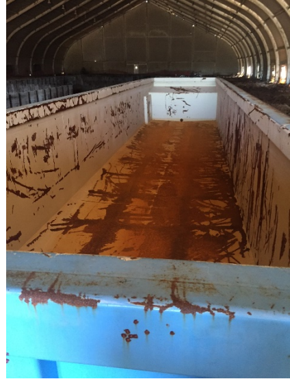
Mix Box located within IB Structure
