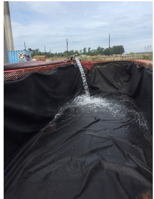
Dewatering activities through vac box
