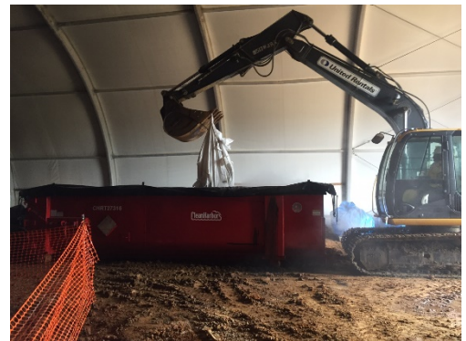
Solidification activities in rolloff box
