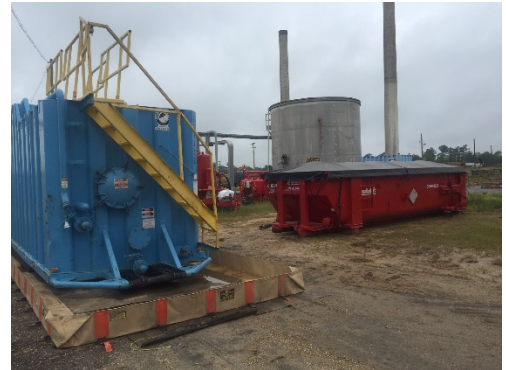
Frac Tank and Rolloff box
