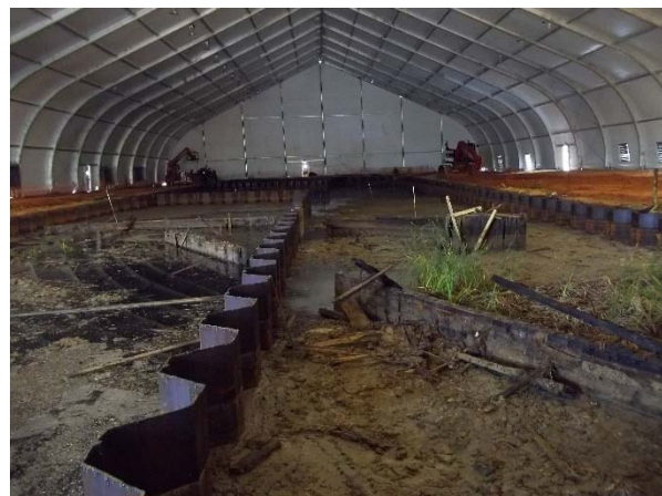
IB during surface water removal activities
