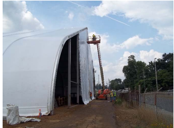
East end wall installation
