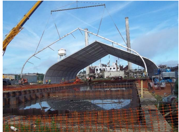
Ongoing truss installation
