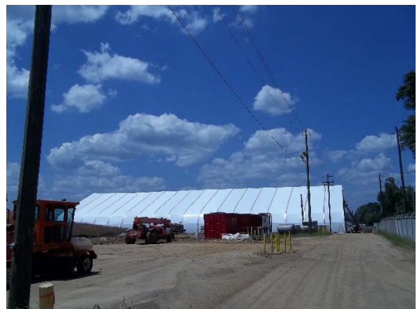
Structure with "skin" installed
