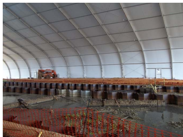
Interior work including lights and air handling equipment
