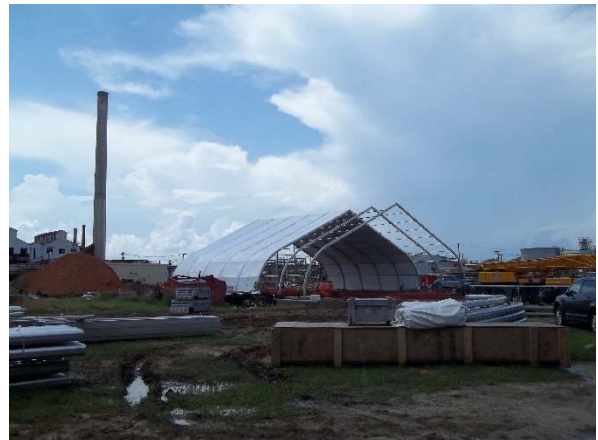
Structure with "skin" installed
