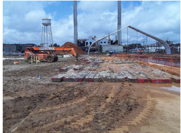
Equipment matting with structure in background
