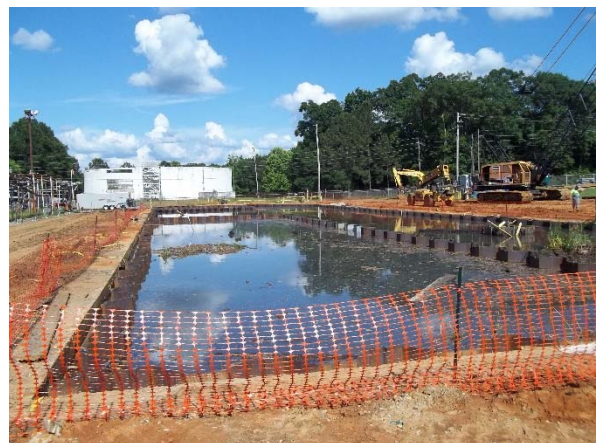
IB with sheet piling at final grade
