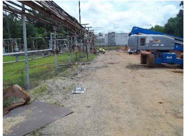
Sprung structure foundation installation
