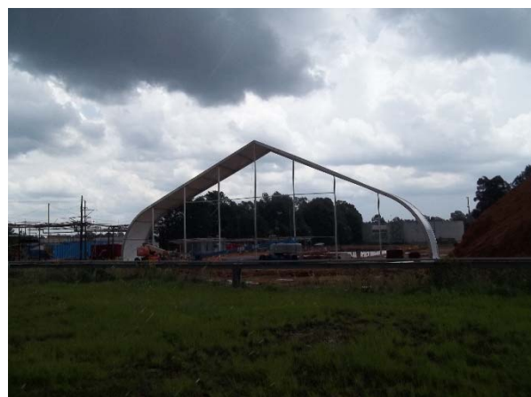
Initial stage of structure construction
