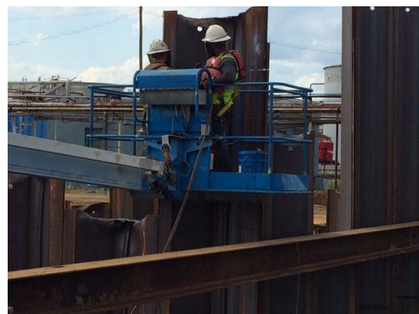
Cutting and removal sheet pile damaged by hammer
