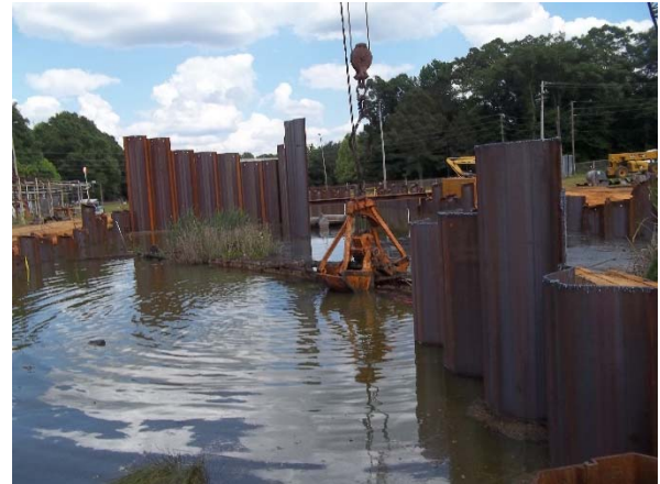
Removal of IB baffles using clam shell bucket
