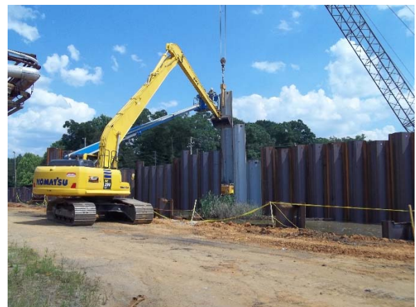
Driving of sheet piles to depth
