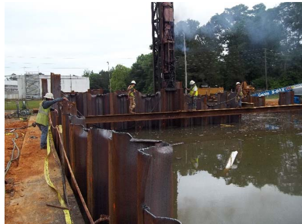
Installation of interior sheet piles
