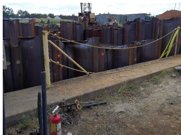
Top of sheet piles bending under pressure from hammer
