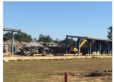
Ongoing facility demolition activities
