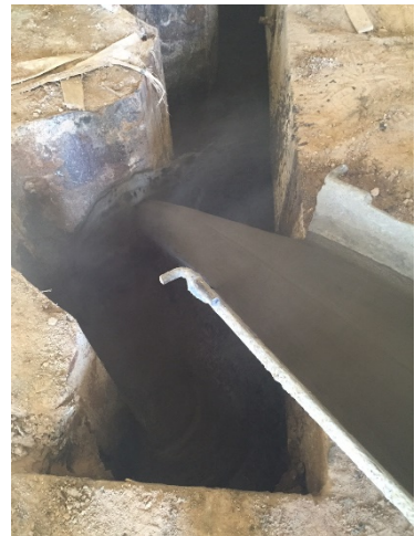
Flowable fill placement in annular space
