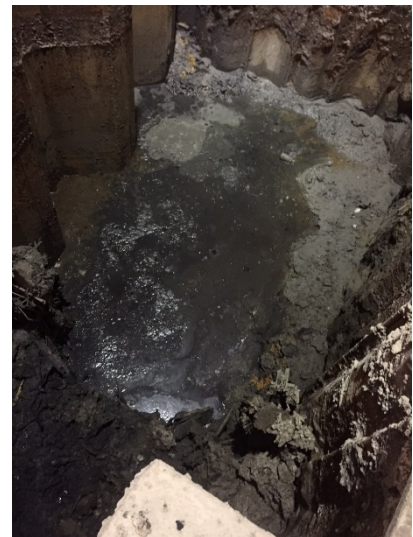
Removal of material from annular ring
