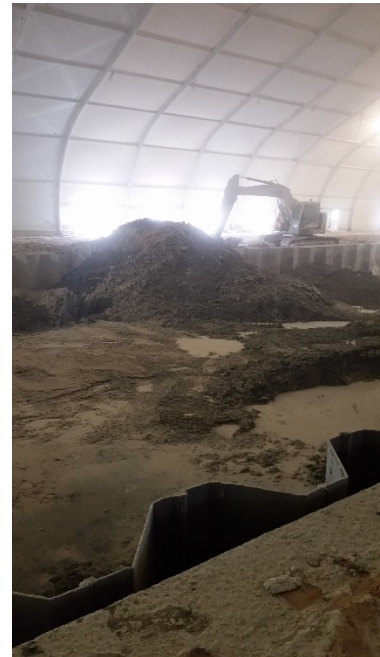
Material mixing and staging
