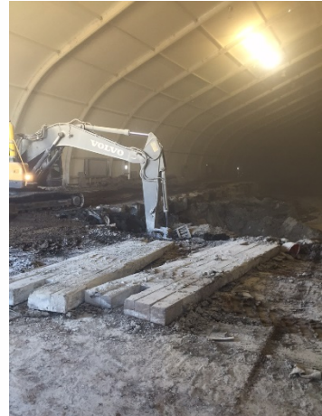
Mixing of material in IB
