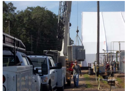
Transformer replacement activities
