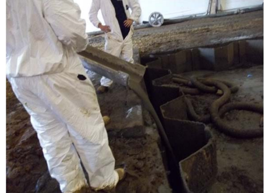
Flowable fill being placed into annular space
