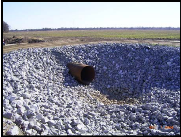
Before and after shots were taken in August and December of 2006 at one location of the Bee Lake Restoration (Holmes County) Project. A rock lined apron was used to prevent scour and erosion at this location.
