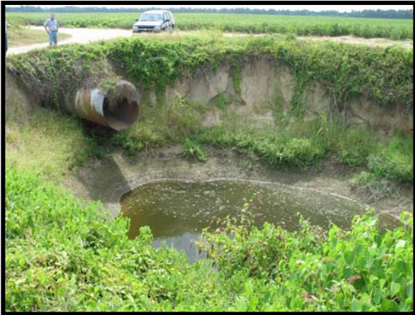
Before and after shots were taken in August and December of 2006 at one location of the Bee Lake Restoration (Holmes County) Project. A rock lined apron was used to prevent scour and erosion at this location.
