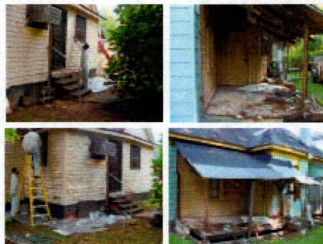
Lead-based paint inspection and removal.
