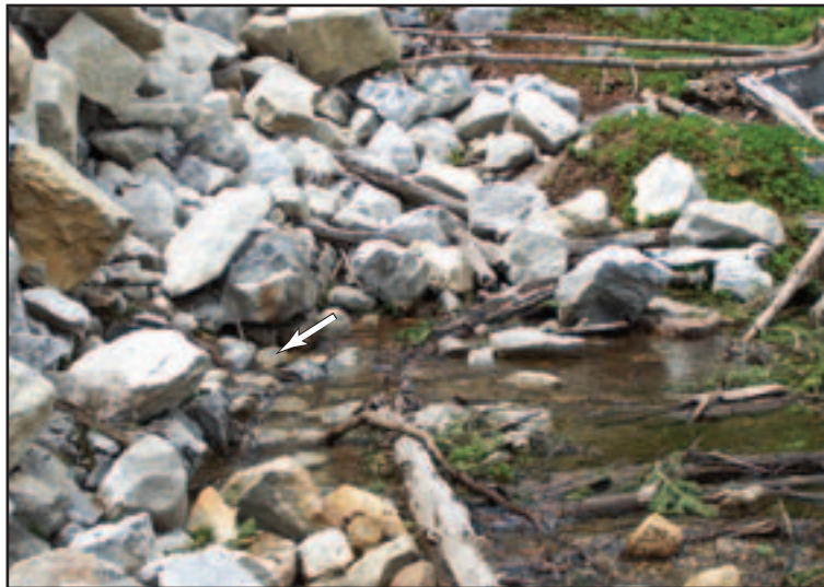
Figure 26—Excessive water piping through the dam at the toe of the embankment.
