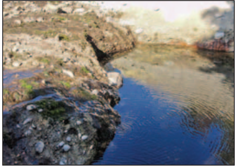
Figure 40—Erosion of the spillway channel may lead to slumps or slides of the spillway sides.
