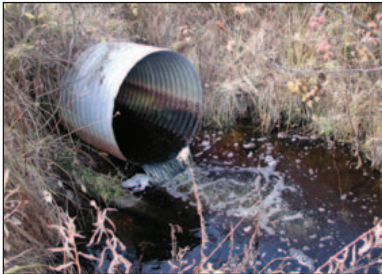
Figure 36—A scour hole at an outlet erodes the toe of the slope.
