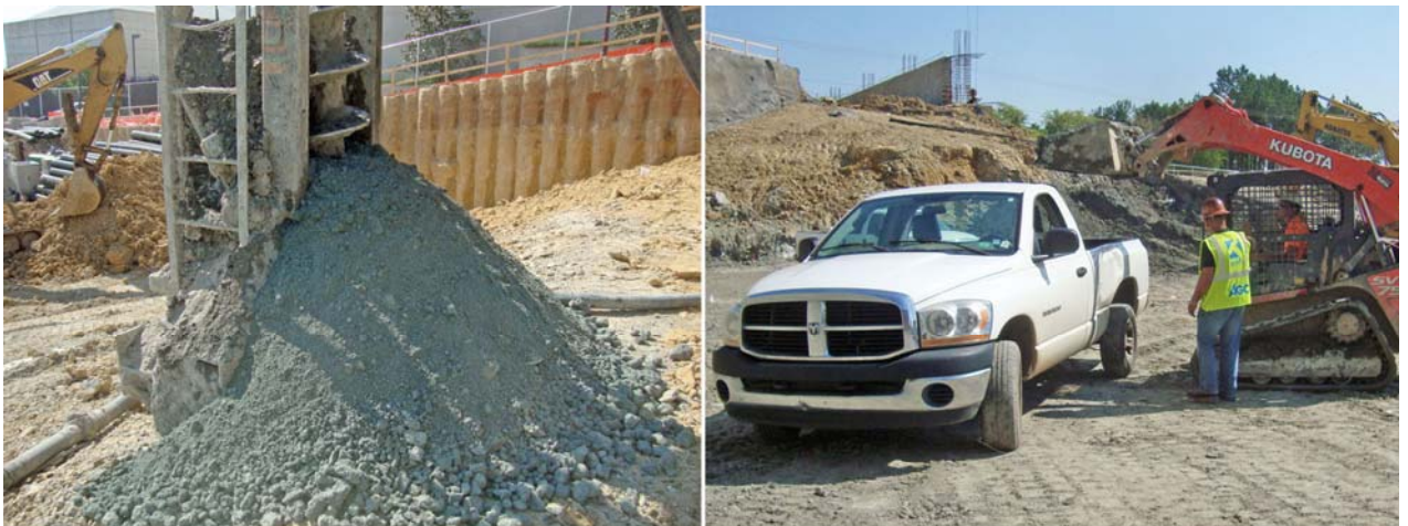
Figure 3. Left: Auger drill hole for pile is bringing up the fossiliferous sands of the Moodys Branch Formation. Right: Front end loader delivers a 1,500-pound load of Moodys Branch Formation sand to a pickup truck. Picture was taken on April 24, 2014.
