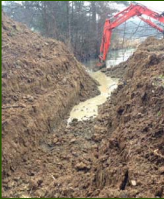
Dam Safety staff supervises the breaching of dams when necessary to protect those downstream.
