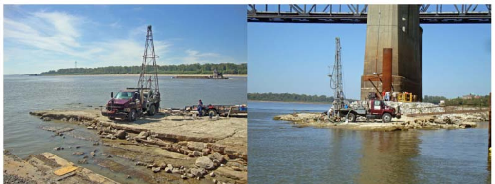
Figure 2. Drilling rig drilling on an island capped by Glendon Limestone in the Mississippi River at Pier E-1 of the Interstate 20 bridge at Vicksburg. At left, the Glendon Limestone plunges below the river level on the south end of an anticline. At right, the vertical pipe behind the rig contains a tiltmeter that measures lateral movement below ground. Pictures were taken on October 15, 2012.
