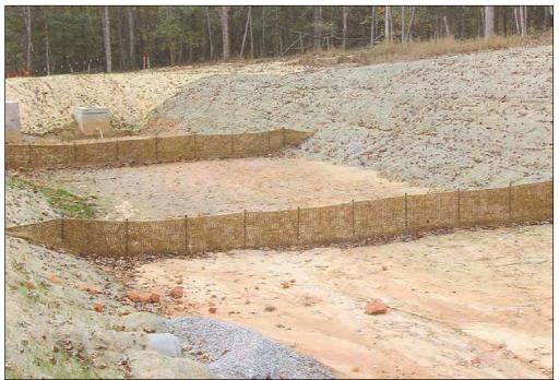
Figure SBN-2 Example of porous baffle made of 700-g/m<sup>2</sup> coir erosion blanket as viewed from the inlet (Source: North Carolina Erosion and Sediment Control Planning and Design Manual)
