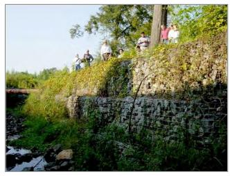
Figure 1: Retaining wall made of gabions
