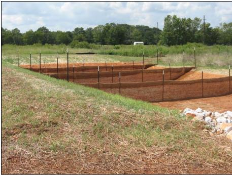
Figure SBN-3 Example of porous baffle made of 700 g/m<sup>2</sup> coir erosion blanket as viewed from the inlet
