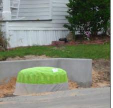
The soil around the drop inlet should be well compacted. The area around the drop inlet should be shaped, if necessary, to store the runoff on an almost level area. If runoff could bypass the protected inlet, a temporary dike should be planned and force the runoff to be trapped by the protective device.
