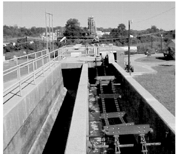
NON-AERATED HORIZONTAL FLOW GRIT CHAMBER
