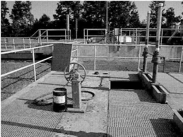
MISSING GRATE AND HOSE ON WALKWAY
