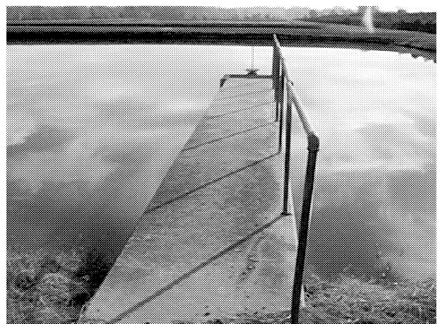
MISSING HANDRAIL ON EFFLUENT STRUCTURE
