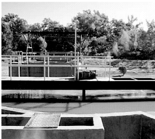
NON-AERATED CIRCULAR FLOW GRIT CHAMBER
