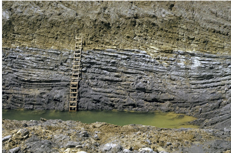
Figure 8. Moodys Branch Formation and Yazoo Clay exposed at sewer excavation (MGS locality 7). Counting ladder steps, the Moodys Branch-Yazoo Clay contact is the 5th step above the water. The upper Yazoo Clay is weathered to a brown color. Picture has a process date of May 1974.
