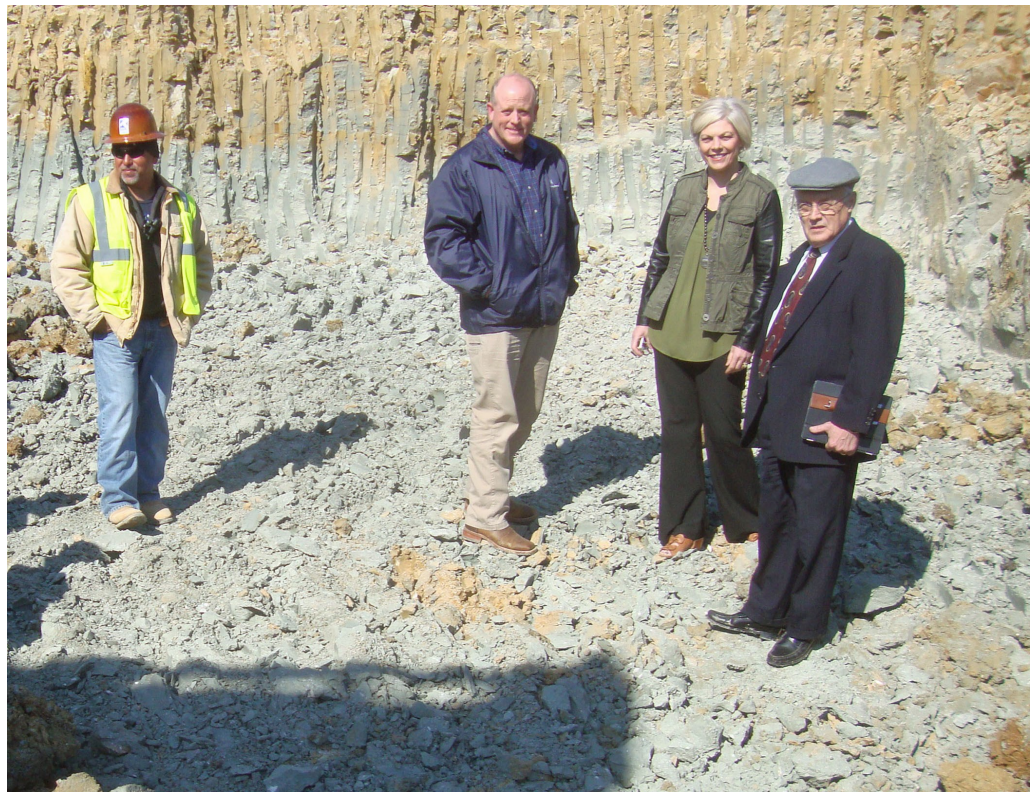
Figure 1. Fossiliferous Yazoo Clay at the construction site of the Museum of Mississippi History. The gray clay at bottom is unweathered and contains chalky fossil shells; above this is brown weathered clay with a potential to swell and shrink. From left to right are Richard Horton (Thrash Commercial Contractors), John Sprayberry (Bureau of Buildings), Sherri Hilton (Director of Communications, Department of Finance and Administration), and Rick Snowden (Deputy Executive Director, Department of Finance and Administration). Picture was taken on March 26, 2014.
