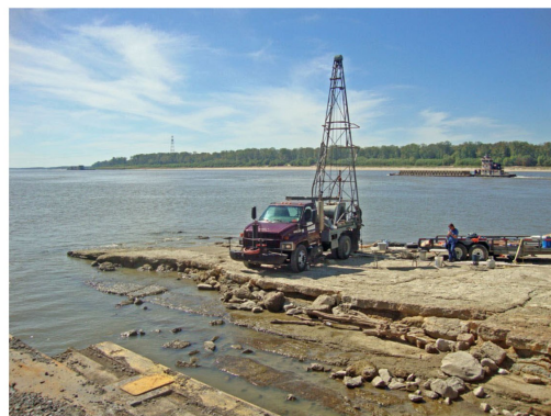
Figure 2. Drilling rig drilling on an island capped by Glendon Limestone in the Mississippi River at Pier E-1 of the Interstate 20 bridge at Vicksburg. At left, the Glendon Limestone plunges below the river level on the south end of an anticline. At right, the vertical pipe behind the rig contains a tiltmeter that measures lateral movement below ground. Pictures were taken on October 15, 2012.
