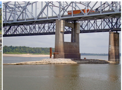
Figure 1. Left: Exposure of Glendon Limestone on the east bank of the Mississippi River beneath the Interstate 20 bridge at Vicksburg. Right: An island of Glendon Limestone in a laterally displaced and down-thrown block, rising out of the river on the south (left) end and plunging beneath the water on the north end in front of Pier E-1 of the I-20 bridge. Here the top ledge of limestone in the adjacent river bank reappears as a doubly plunging anticline. Picture on left was taken on October 15, 2012, and the picture on the right was taken on August 14, 2012.
