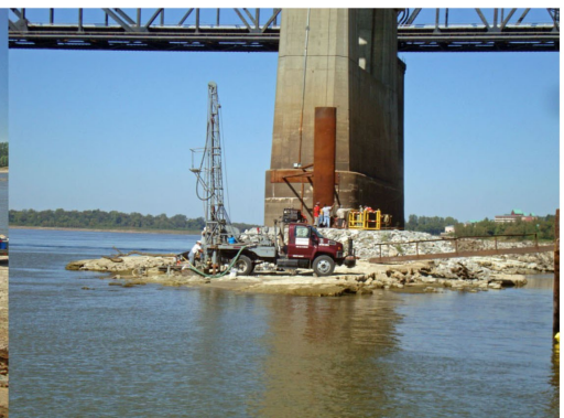
Figure 2. Drilling rig drilling on an island capped by Glendon Limestone in the Mississippi River at Pier E-1 of the Interstate 20 bridge at Vicksburg. At left, the Glendon Limestone plunges below the river level on the south end of an anticline. At right, the vertical pipe behind the rig contains a tiltmeter that measures lateral movement below ground. Pictures were taken on October 15, 2012.
