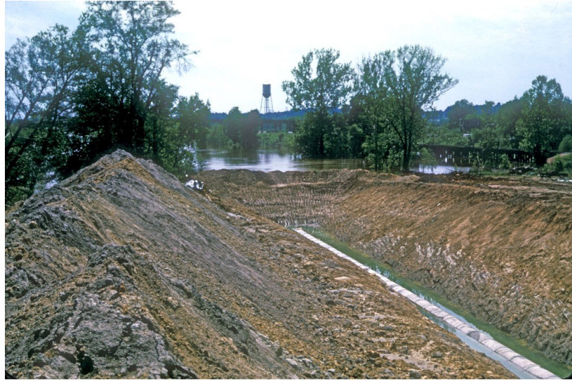
Figure 7. Sewer excavation and pipe on the north bank of Town Creek. Spoil berms serve as levees to keep out the flood waters of the Pearl River. Picture has a process date of May 1974.
