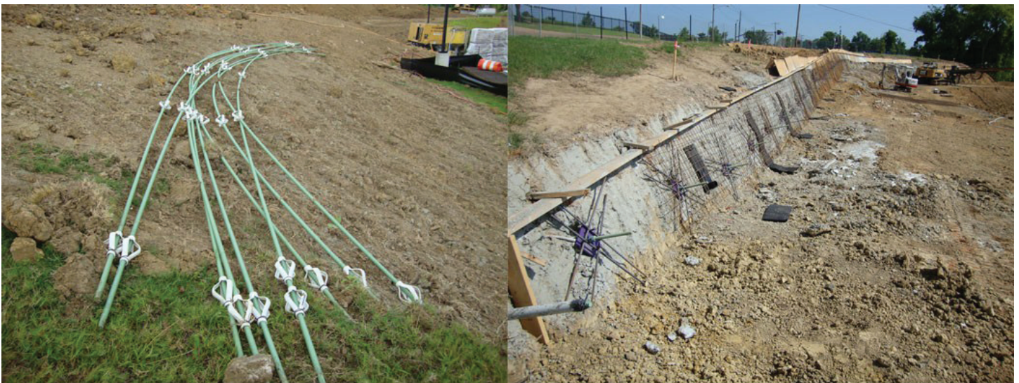
Figure 3. Left: Rebar and spacers for soil nails. Right: Forms, grouted rebar (soil nails), and welded wire mesh of the upper tier of the Farmer's Market retaining wall. Pictures taken on July 28 (left) and July 31, 2010. (Image 1683)
