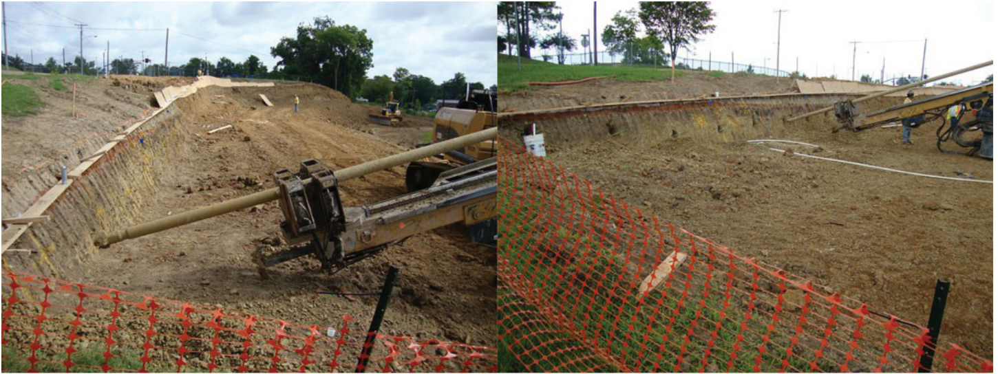
Figure 2. Left: The yellow cross marks the spot for drilling the hole for the second soil nail in the upper tier of the Farmer's Market retaining wall. Right: Rebar protrudes from five holes, while a sixth hole is being reamed out. The white hose is for pumping grout. Pictures taken on July 28, 2010. (Image 1682)
