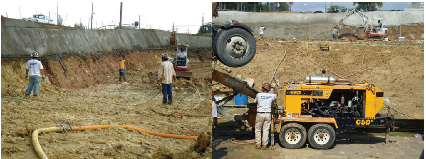
Figure 5. Left: Workers hurry to insert rebar into drill holes in the south end of the middle tier after an afternoon storm sends water pouring in from behind the wall at the contact of brown Yazoo Clay and red fill dirt just to the right of the man at far left. A leak in a 6-inch city water main was discovered, which contributed to the flow; the leak was repaired by the city that evening. Right: Cement truck pours shotcrete into hopper where it is pumped through a hose and sprayed onto the soil nails and welded wire mesh on the troubled south end of the middle tier to seal the leak site behind the Farmer's Market retaining wall. Pictures taken on August 4 (left) and August 6, 2010 (right). (Image 1685)
