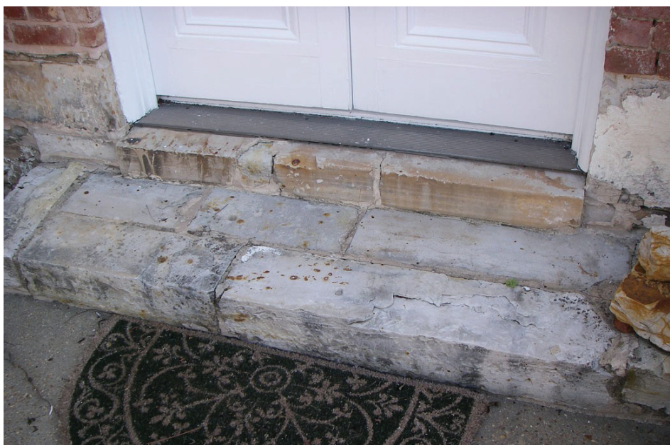
Figure 2. Catahoula sandstone steps and facing/foundation stones in a building on the Raymond town square. Picture (digital) taken on September 20, 2007.
