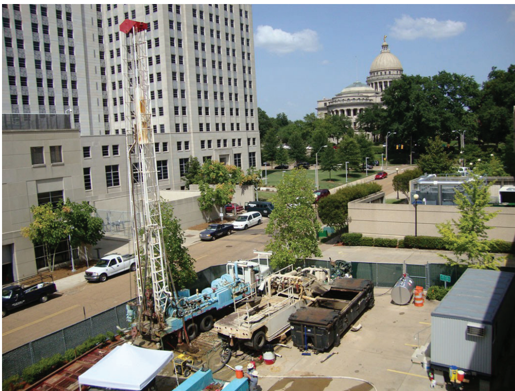
Figure 7. Drilling of an eight-hundred-foot-deep well in the Sparta aquifer by the Donald Smith Company for the Mississippi Department of Transportation. Picture (digital) taken on July 22, 2010.
