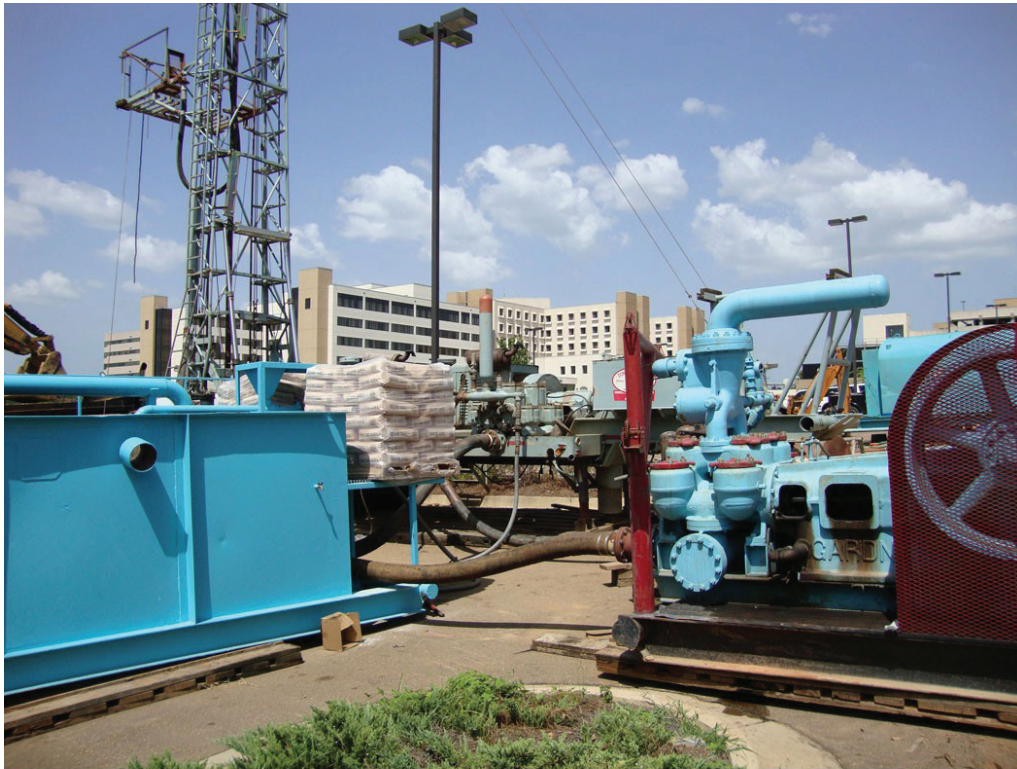
Figure 6. Drilling of an eight-hundred-foot-deep well in the Sparta aquifer by Donal Smith Company for the Baptist Hospital. Picture (digital) taken on June 22, 2010.
