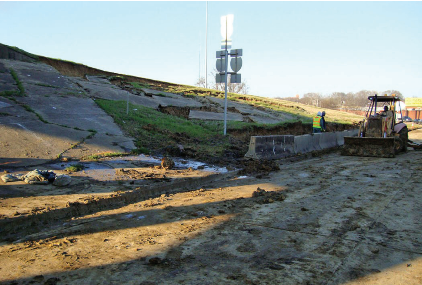
Figure 2. Work crew excavates slump toe from Terry Road at Interstate 20 and erects concrete barriers to keep the toe off the road. Picture (digital) taken on the afternoon of February 9, 2010.
