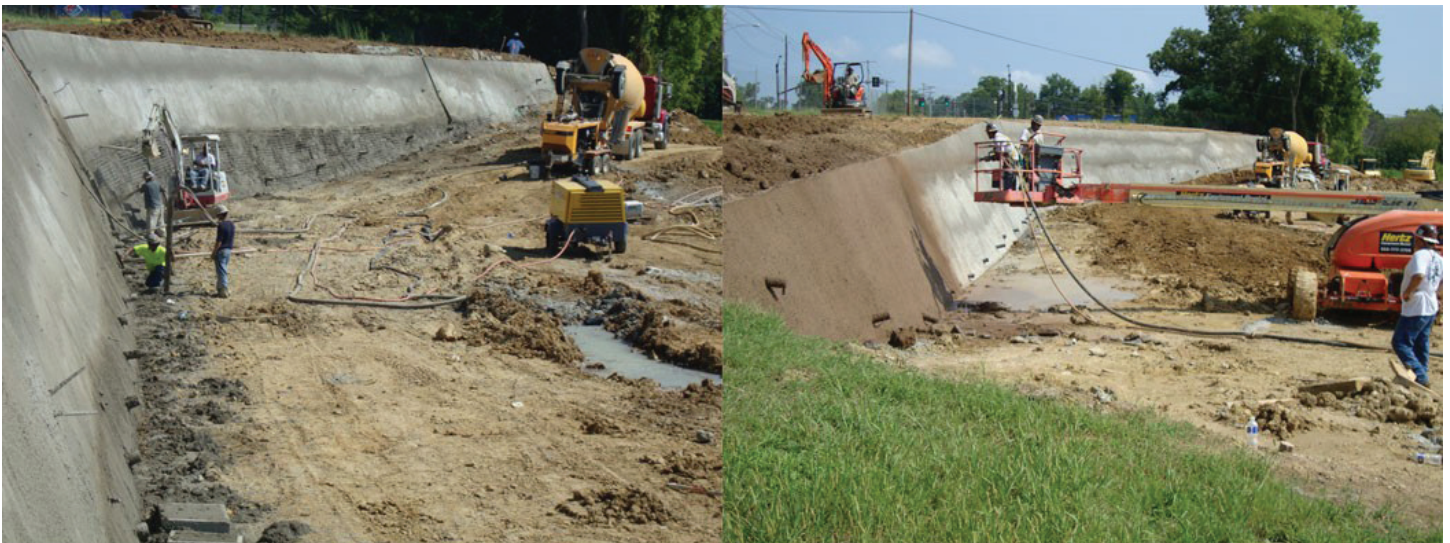
Figure 7. Left: Shotcrete is sprayed onto the welded wire mesh of the lower tier of the Farmer's Market retaining wall. Right: A brown dirt-colored grout is sprayed over the entire retaining wall to give it a natural appearance (like dirt). Water drains can be seen protruding from the base of the wall. Pictures taken on August 12 (left) and August 16, 2010 (right). (Image 1687)
