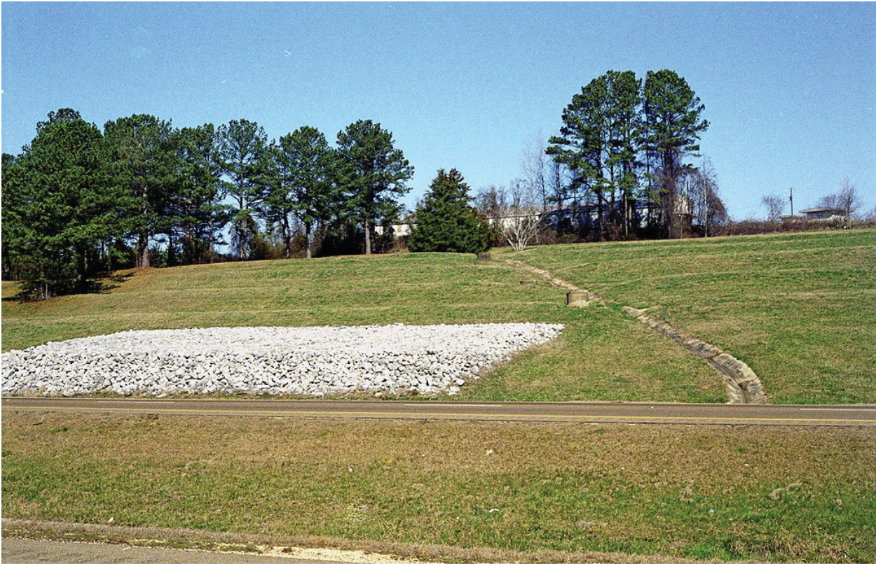
Figure 4. Rip-rap and concrete drain installed to prevent slumping in the Yazoo Clay on a roadcut north of the Interstate 20 west-bound lane near Forest, Mississippi. Picture (color negative 568-0A) taken on March 1, 2006.
