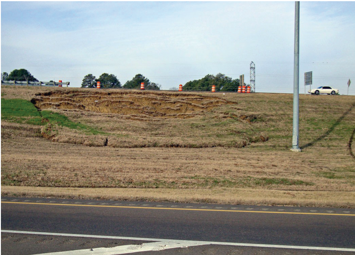
Figure 5. Slump in the Yazoo Clay on the east side of Interstate 220 South near the I-20 interchange. Picture (digital) taken on February 10, 2010.
