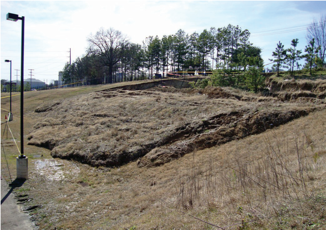
Figure 6. Slump in Yazoo Clay behind the new Farmer's Market. The slump scarp at top threatens a water main and Jefferson Street. Picture (digital) taken on February 18, 2010.
