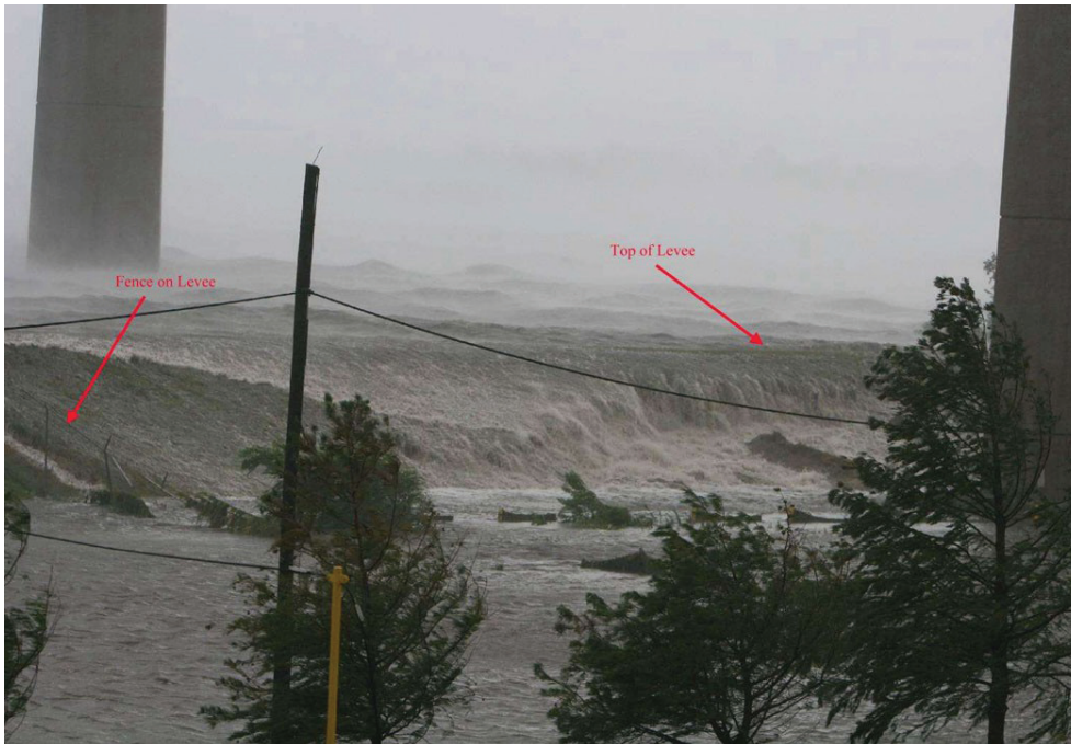
Figure 6. Katrina storm surge with high waves topping the levee on the north side of the Intracoastal Waterway right under the Paris Road/Highway 47 bridge. Picture taken by someone at the Entergy Power Plant in the early morning of August 29, 2005.
