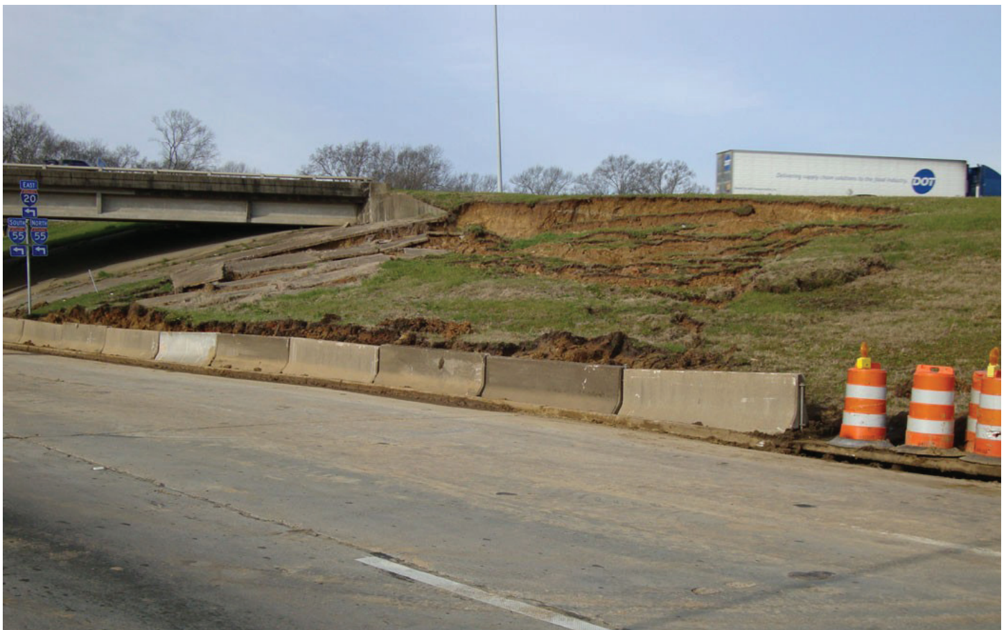
Figure 3. Slump in Yazoo Clay on Terry Road at Interstate 20 in Jackson. Concrete barriers keep the slump toe off the road; the slump has fractured the concrete apron under the I-20 bridge. Picture (digital) taken on February 10, 2010.
