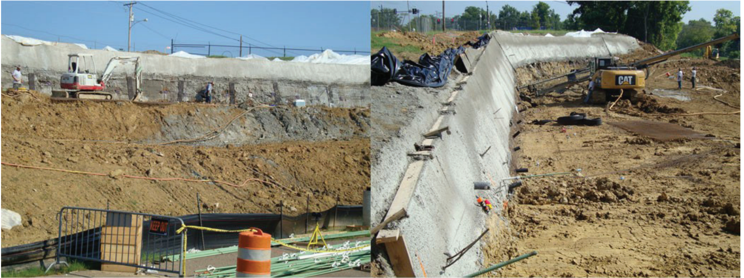
Figure 6. Left: Welded wire mesh is checked before shotcrete is sprayed on the north end of the wall's middle tier. The black vertical strips are drains to prevent the accumulation of water behind the wall. Right: Holes are drilled for the soil nails of the lower tier of the Farmer's Market retaining wall. Drain pipes are visible at the base of the wall. Pictures taken on August 9 (left) and August 11, 2010 (right). (Image 1686)
