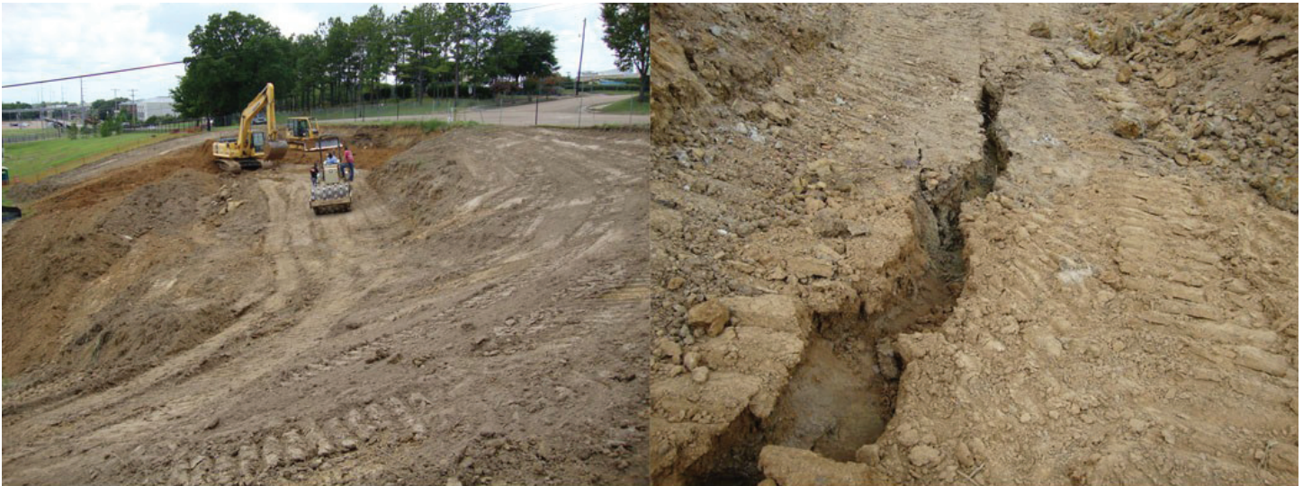
Figure 1. Left: Adding and compacting fill material to the upper slope behind the Farmer's Market on July 19, 2010. Right: New failure in the Yazoo Clay of the upper slope the following day on July 20, 2010. (Image 1681).
