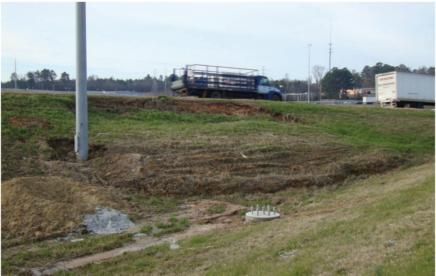
Figure 1. Slump in Yazoo Clay on the north side of Interstate 20 west of Gallatin Street. Picture (digital) taken on February 10, 2010.
