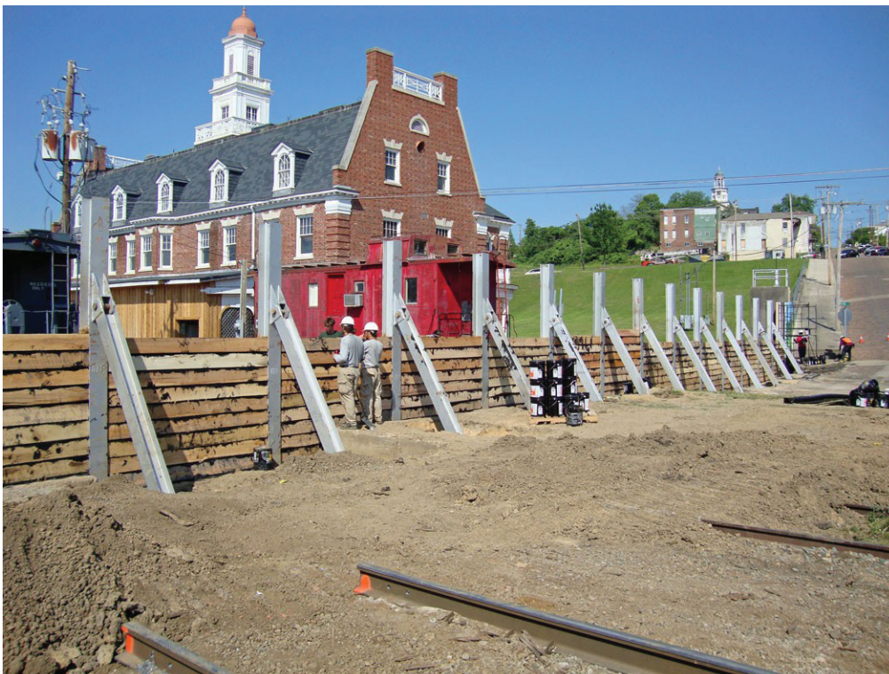
Figure 5. Planking up and tarring the north end of the Vicksburg flood wall. Picture was taken on May 6, 2011.
