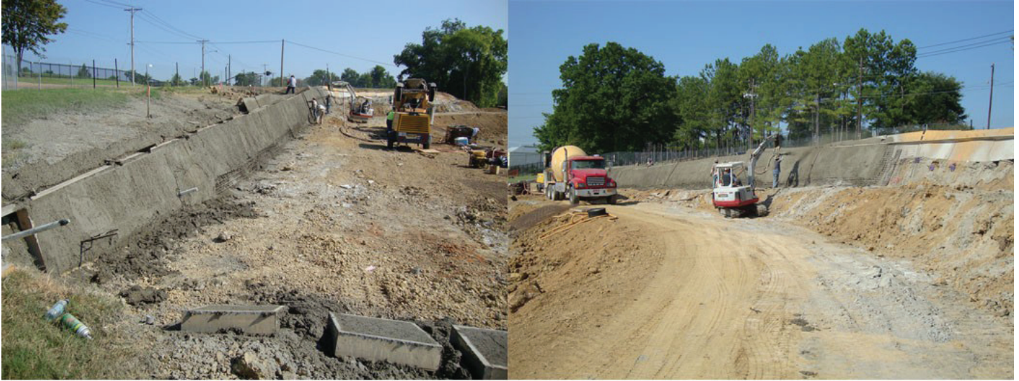
Figure 4. Left and right: Spraying shotcrete onto the welded wire mesh of the upper tier of the Farmer's Market retaining wall. Pictures taken on August 2, 2010. (Image 1684)
