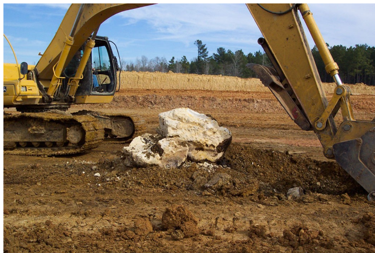
Figure 2. Backhoe excavating pinnacles of limestone, at the request of MDEQ geologists, from swelling clays in the Glendon regolith under the graded foundation for the new Brandon High School. This soil proved unsuitable as foundation material and was removed at a considerable cost overrun. Picture (digital CD #44) taken by Stephen Jennings on January 28, 2004.
