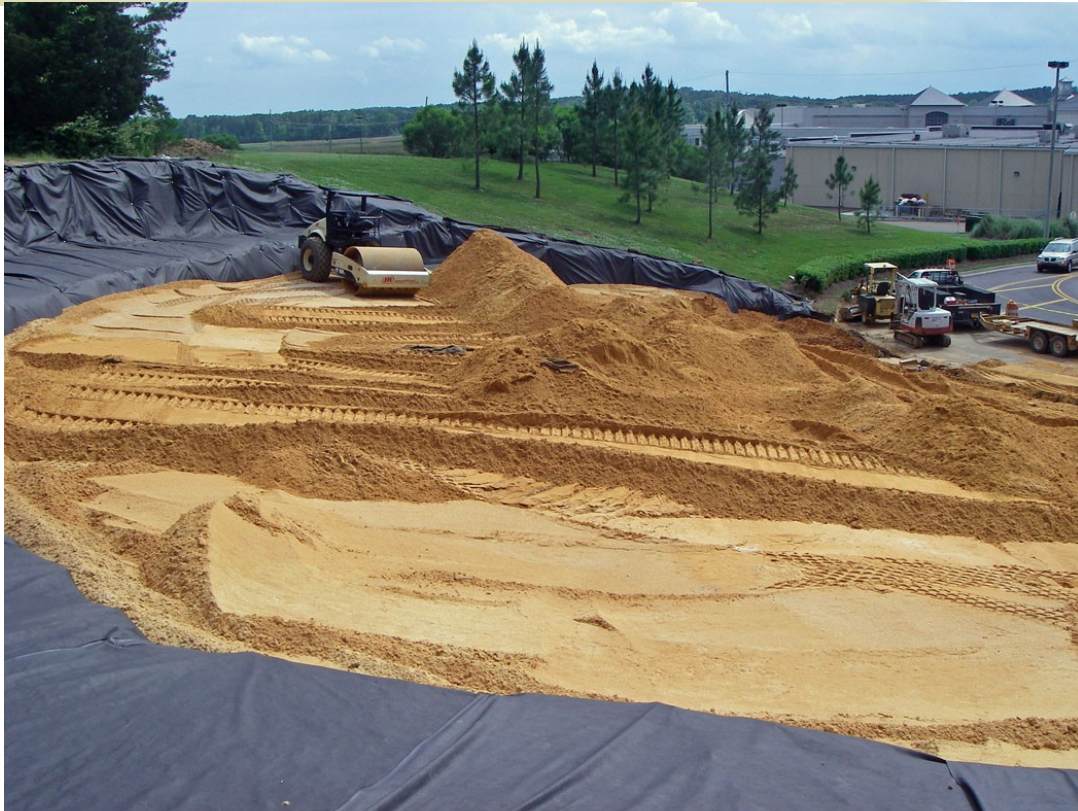
Figure 4. Slump excavation is sealed in fabric and backfilled and compacted with a 96 % pure grade of sand. Dogwood Festival can be seen in the upper right. Picture (DVD #59) taken on May 1, 2009.
