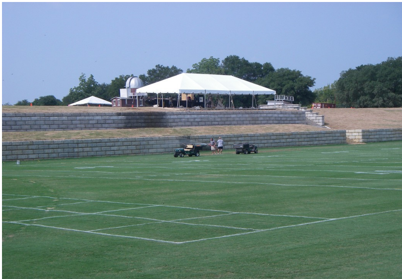
Figure 7. New retaining wall at Millsaps College completed in time for the Saints' summer football camp. The upper wall was extended from 205 to 300 feet to the east (left) of the stairs.
