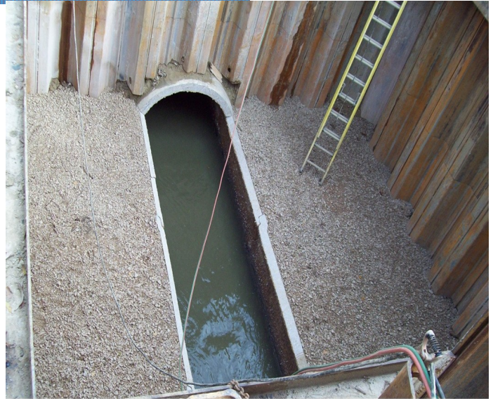
Box cut to the Jackson sewer line near the east end of Rankin Street adjacent to Town Creek. The line was cut at 10 o'clock and 2 o'clock to insert a liner that will protect the concrete pipe from the corrosive effects of sewer gas. The picture (digital) was taken by James Starnes on December 5, 2008, a time of low water on the Pearl River.
