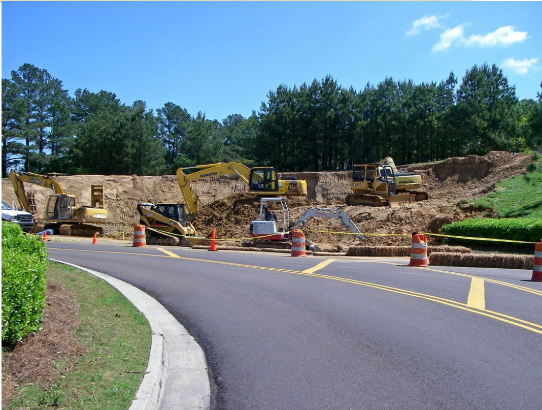
Figure 2. Excavation of slump on the east side of the east entrance to Dogwood Festival on Highway 25 in Flowood, Mississippi. Picture (digital CD #59) taken on April 20, 2009.
