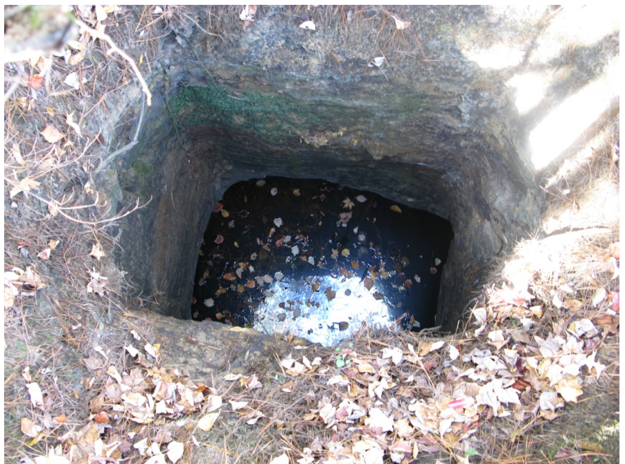
10' x 11' x 23' deep flooded vertical air shaft near Ackerman, Choctaw County
