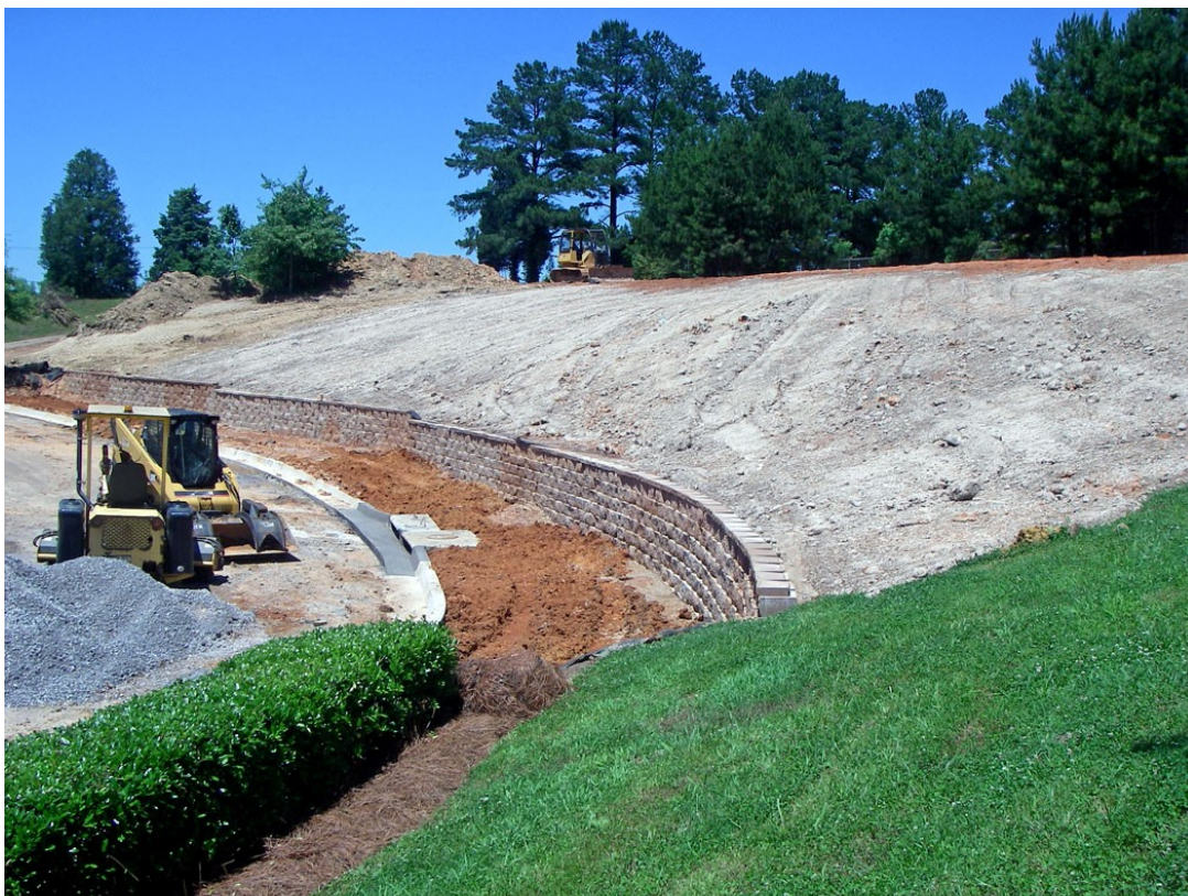
Figure 5. Slump repair near completion with the storm drain repaired, the retaining wall in place, and the sand fill covered with fill dirt. Picture (DVD #59) taken on May 18, 2009.
