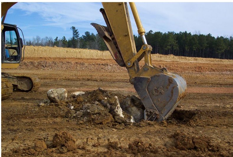
Figure 1. Backhoe excavating pinnacles of limestone, at the request of MDEQ geologists, from swelling clays in the Glendon regolith under the graded foundation for the new Brandon High School. This soil proved unsuitable as foundation material and was removed at a considerable cost overrun. Picture (digital CD #44) taken by Stephen Jennings on January 28, 2004.
