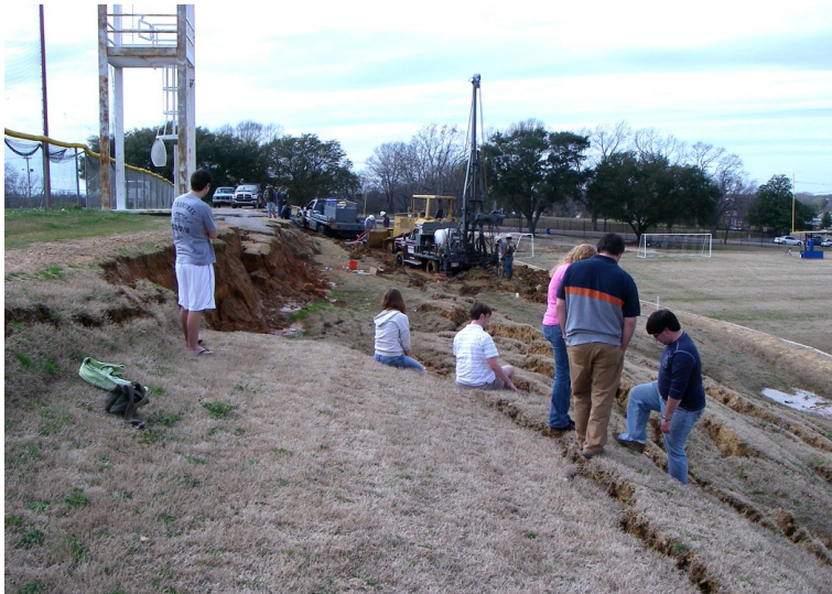
Figure 3. Millsaps geology students watch as an auger rig drills a hole to determine the base of the slump block adjacent to the new football field at Millsaps College. Picture (digital CD #42) taken on February 20, 2008.
