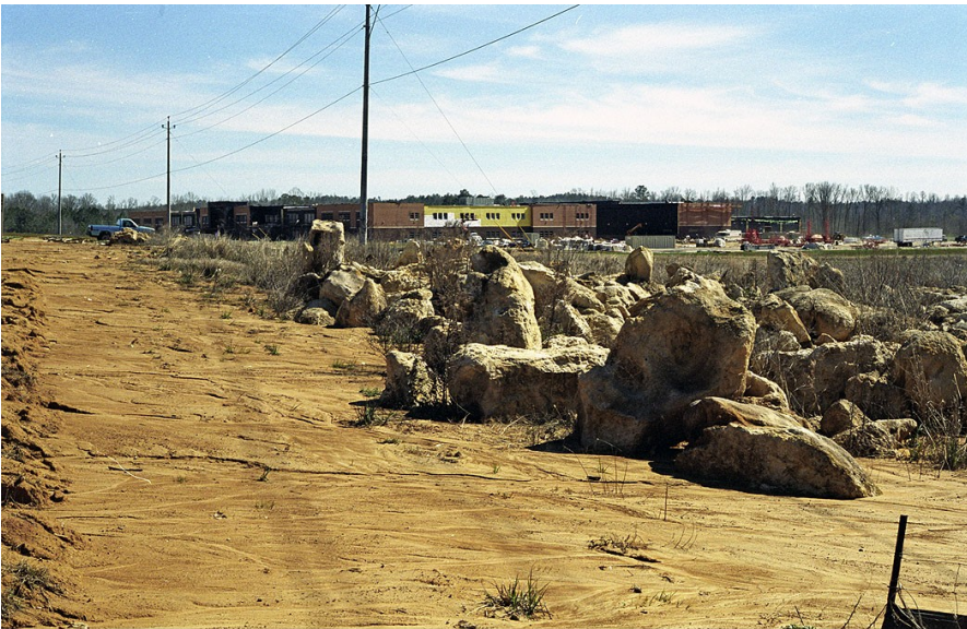
Figure 3. Boulders of Glendon Limestone excavated from the site of the new Brandon High School where foundation problems were found associated with the weathered limestone. Picture (color negative 540-23A) taken on March 8, 2005.
