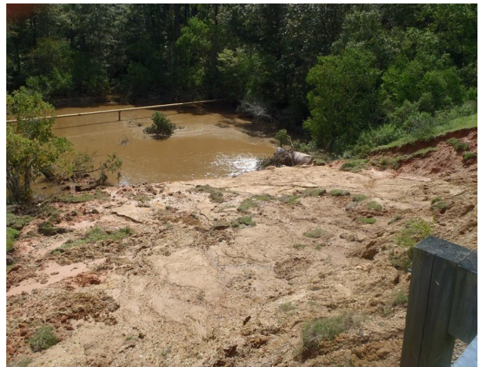
Landslide on the Percy Quin State Park dam caused by Hurricane Isaac
