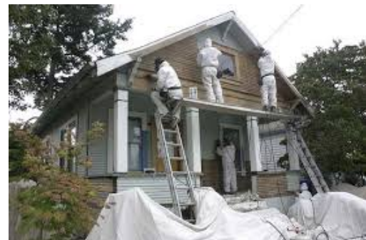
Lead-Based Paint Renovation Project
