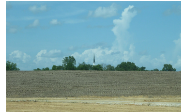
East Containment Cell (prior to seeding)
