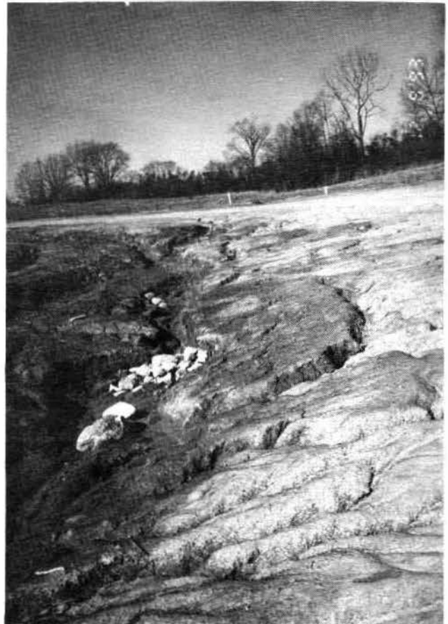
Figure 2. Construction site showing extensive soil erosion due to rain runoff.
