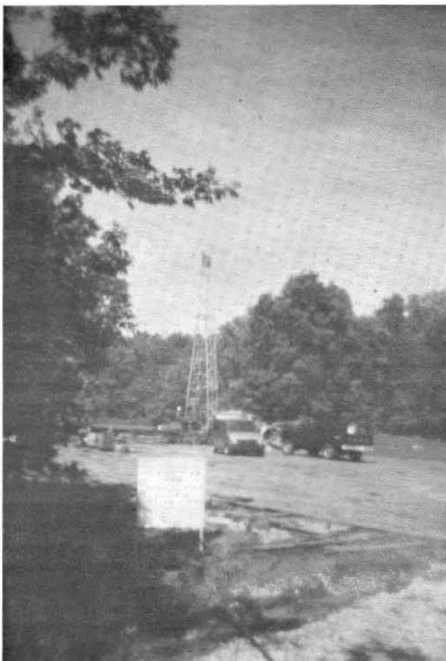
Figure 2. The Plantation Petroleum Company, No. 1 Allen, core hole drillsite and Longyear core hole drilling rig.
