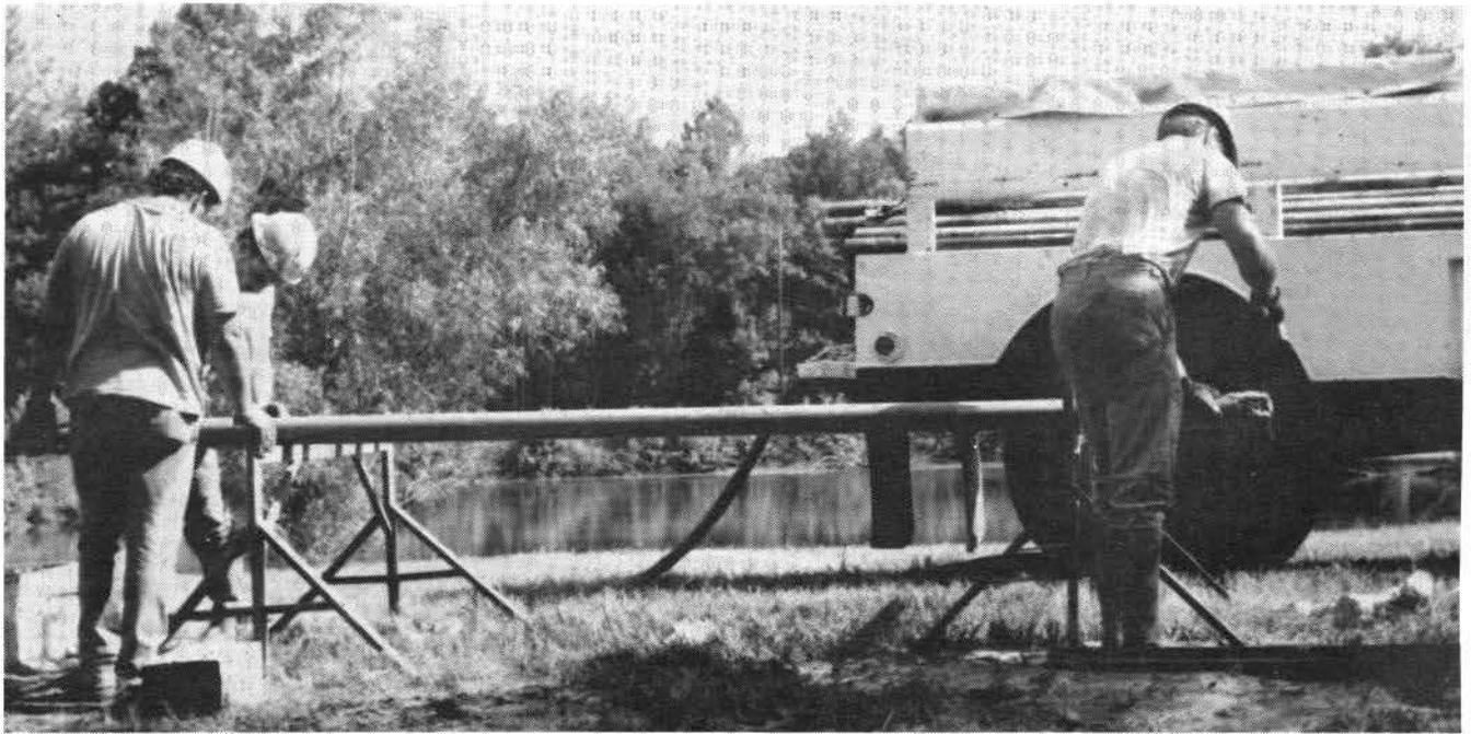
Figure 5. Breaking the bit loose from the core barrel (at right) and inserting the mud hose into fitting (at left).
