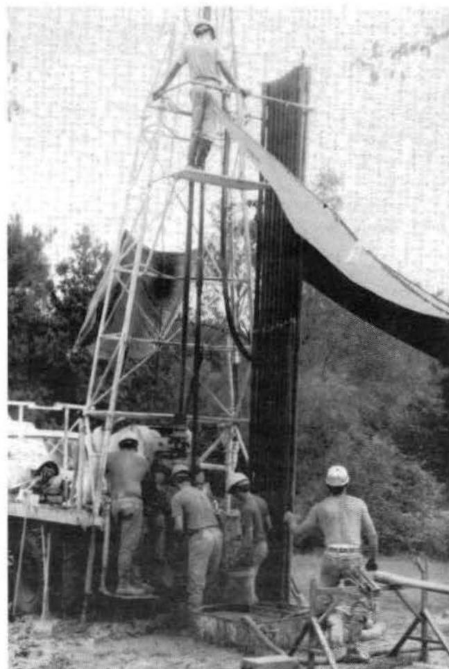
Figure 4. Bringing the core out of the hole with 17 20-foot sections stacked against the monkey board and another being broken from the drill stem at the breakout table. Phillip Weathersby is on the monkey board (top) and on the ground from left to right are Scott Mixon, Wayne Stover, Archie McKenzie, and Steve Ingram.
