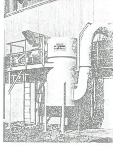
ROUND SCRUBBER—Sealed Power Corp. Vents spin molding machines. Built to operate at 5,000 CFM, 120°F, the scrubber has provisions for increasing capacity to 6,000 CFM.
