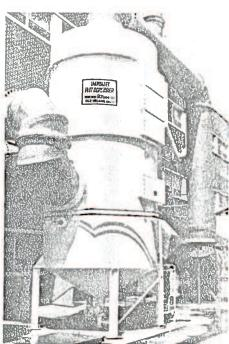
ROUND SCRUBBER — Sylvania Electric Products, Inc. This three stage IMPINJET is used for dust control and furne absorption. The unit is designed to handle 30,000 CFM at 180°F. Polyvinyl dichloride (PVDC) impingement baffle plates and butyl lined shell are employed to resist corrosion.
