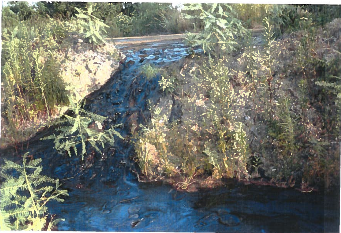
Photo № 19 Roll № 1 Frame №: 20 Date: 6/25/92 Subject: Sludge flow through a breach in the containing dike. Near the E-0 tank.
