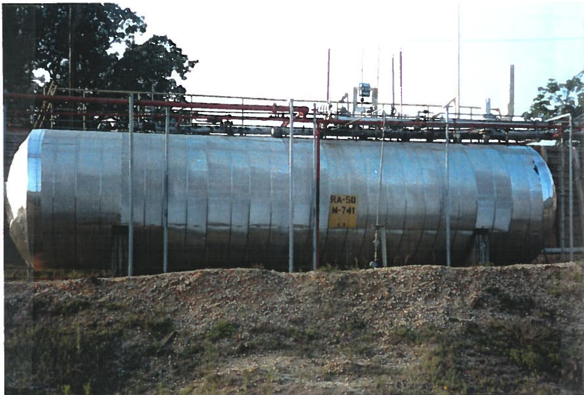
Photo № 17 Roll № 1 Frame №: 18 Date: 6/25/92 Subject: The E-0 Tank (Ethylene Oxide) located in the northeast portion of site property.
