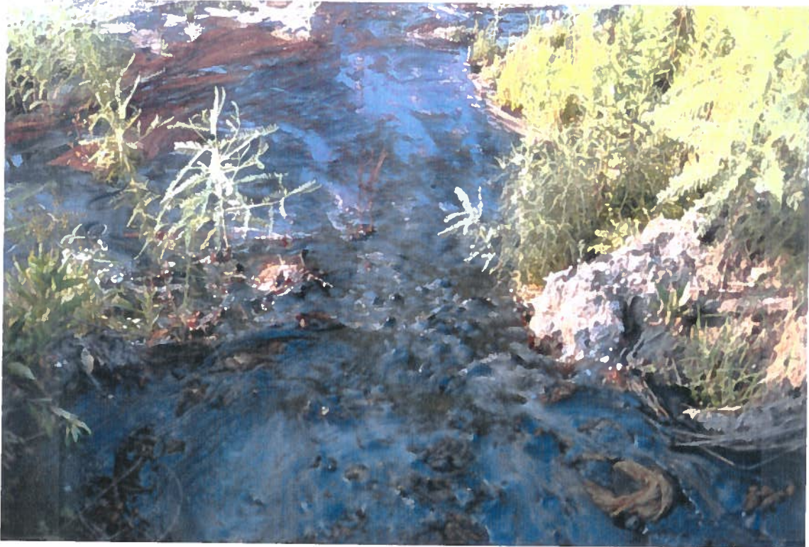
Photo № 14 Roll № 1 Frame №: 15 Date: 6/25/92 Subject: A dike breach in the sludge pits located near the E-0 tank, northeast corner of site property.
