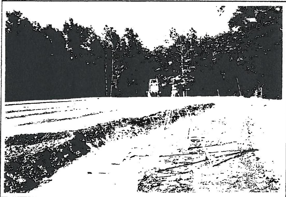
PHOTO 15: 350D Dozer Grading Drainage Layer
