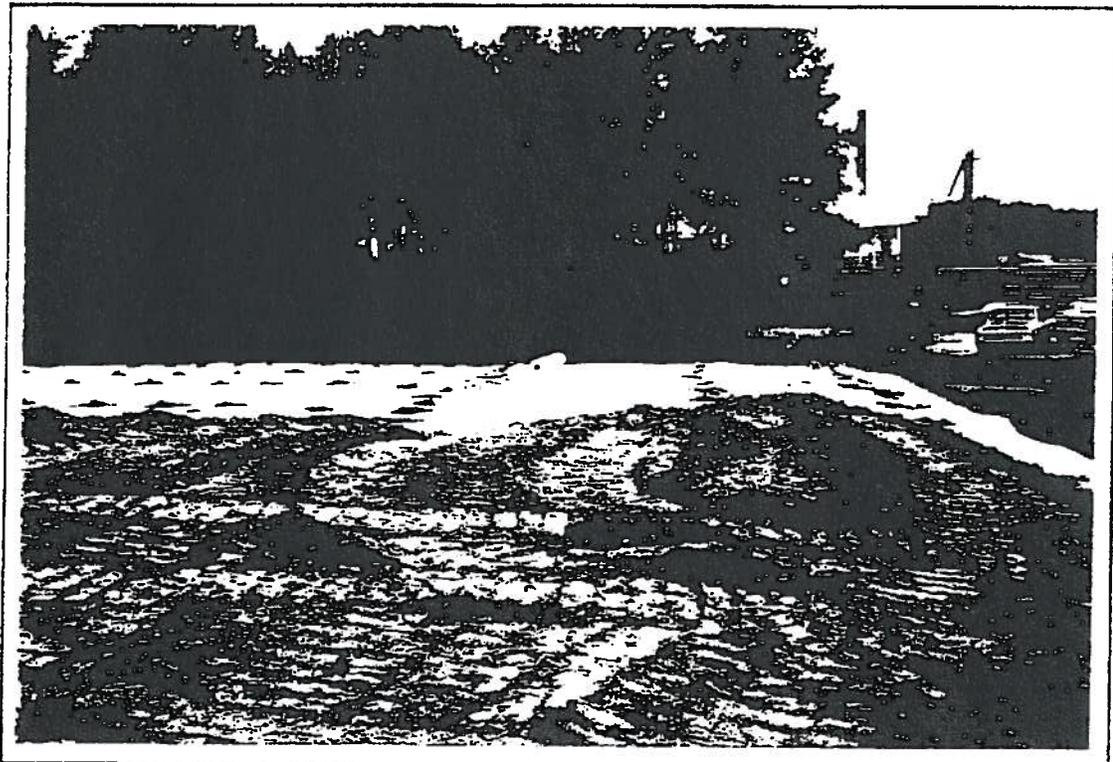
PHOTO 20: Placing Filter Fabric onto Drainage Layer and Pushing Cover Soil onto the Fabric
