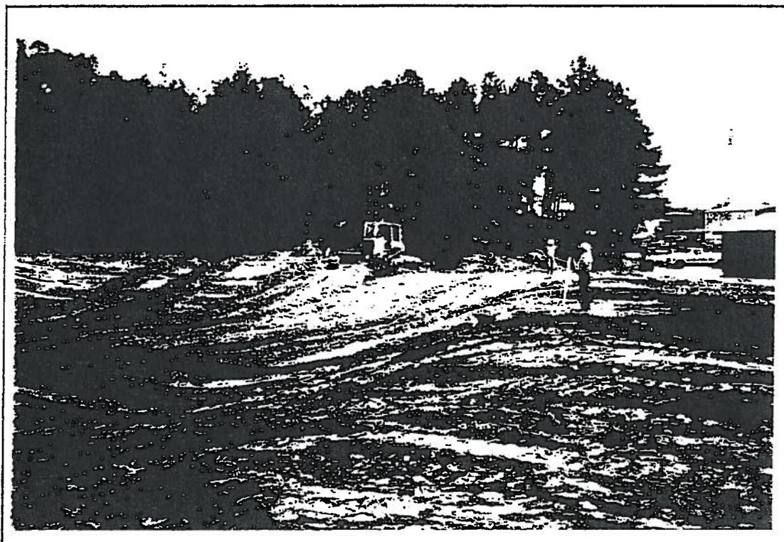
PHOTO 4: Checking Grade Elevation During Cut and Fill
