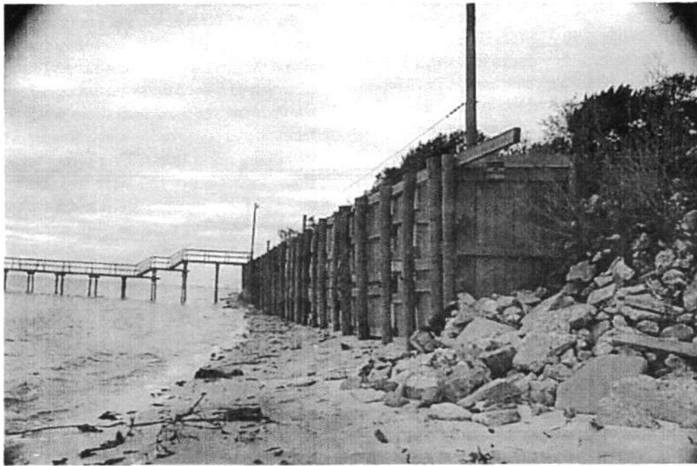
Figure 2. This large bulkhead is to the east of the study area and was constructed directly on the Gulfport Formation cliffs. This cliff is a major source of sand, which has been blocked off, for the beaches of the study area.
