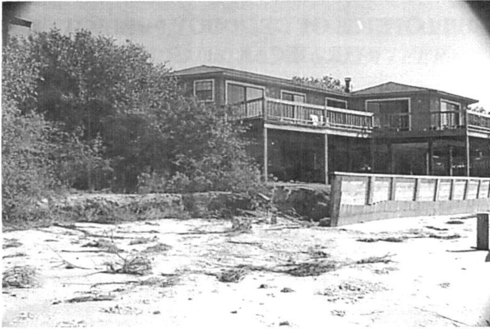
Figure 7. Before the storm event occurred, all properties in the area had bulkheads. The Seymour family had a strong, well-built bulkhead, while their neighbors to the left and right completely lost bulkheads and had property damage (notice scarps to the left of the picture).
