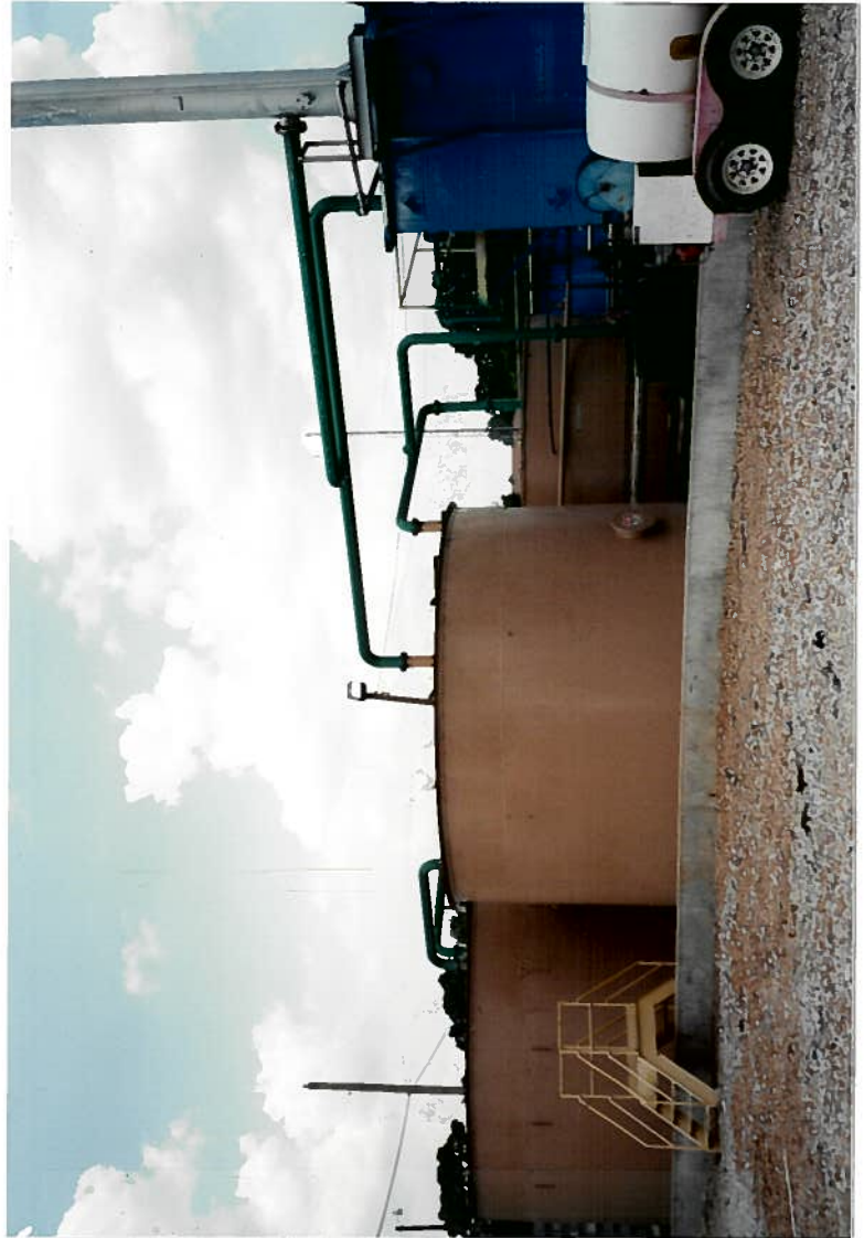
Photo 4 - Settling Tanks and Oil/Water Separator with Vent Stack
