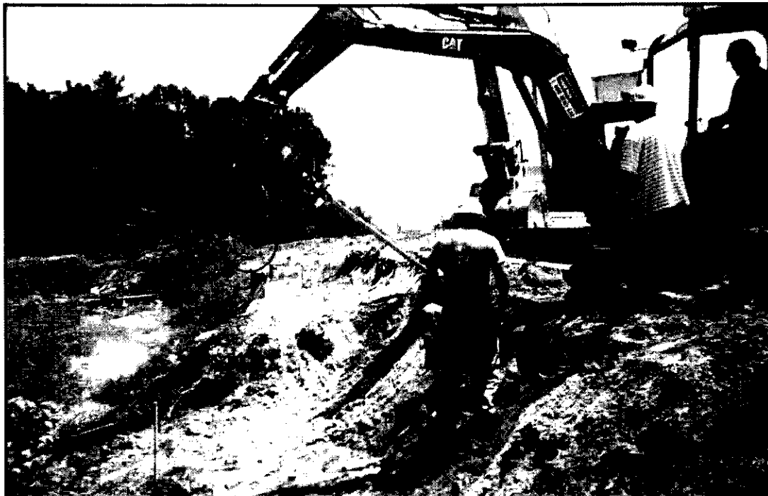
Photo 7.9: Typical Tieback Installation
