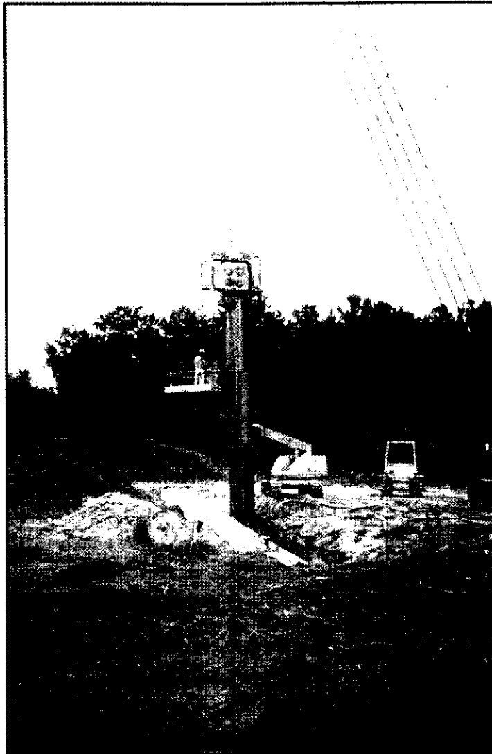
Photo 7.2: Sheet Pile Driving
