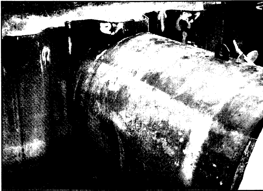
Photo 7.4: Continuous Weld Around the Penetration
