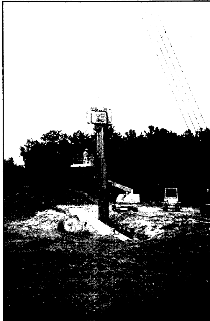
Photo 7.2: Sheet Pile Driving
