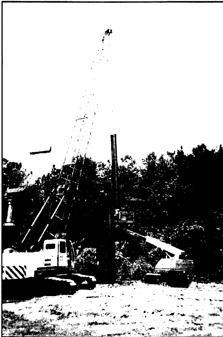
Photo 5.2: Pile Driving Equipment - General Setup
