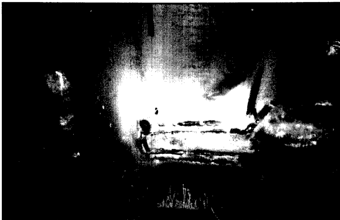
Photo 7.7: Continuous Weld along Pipe Penetration
