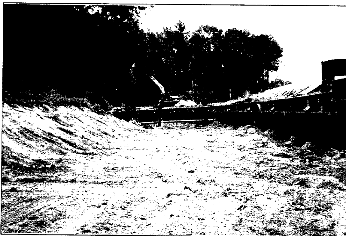
Cleaned and re-graded channel of Gordon's Creek
