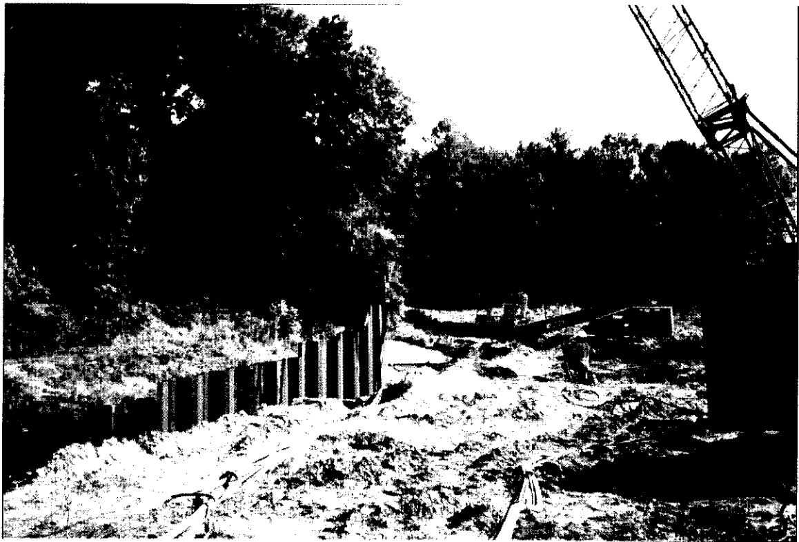
Driving piles along Gordon's Creek (facing north)
