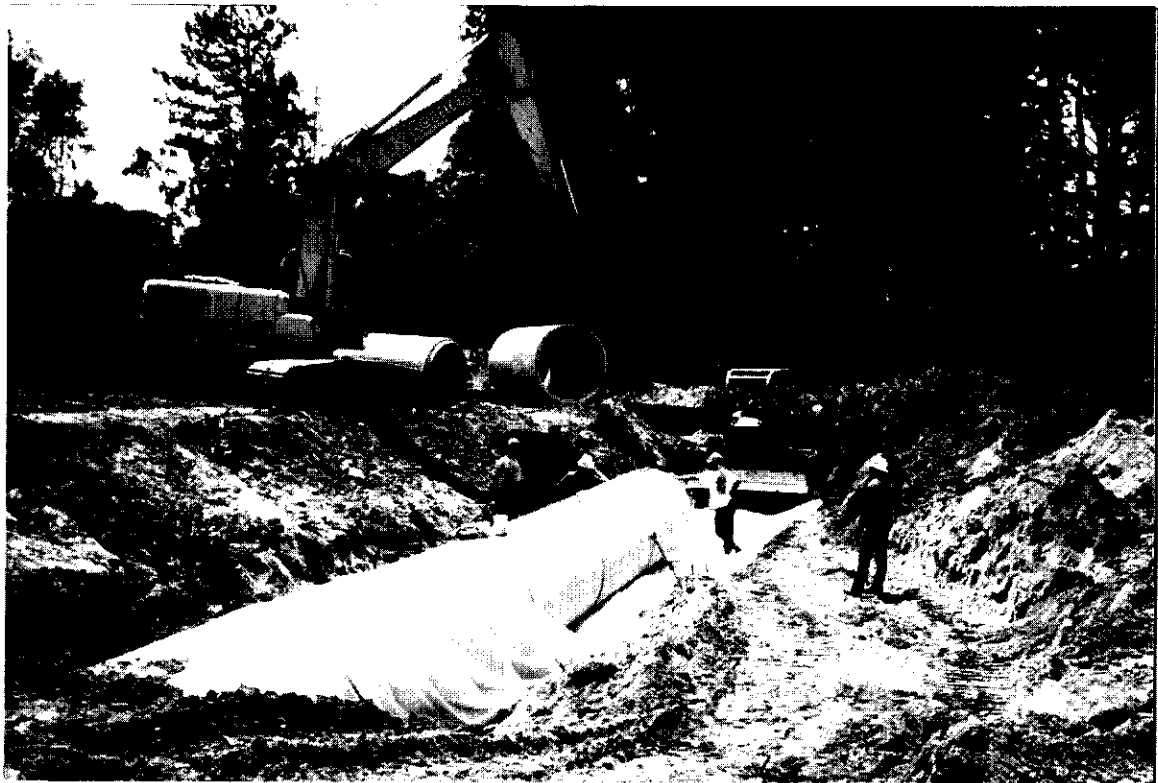
Fill Area culvert installation
