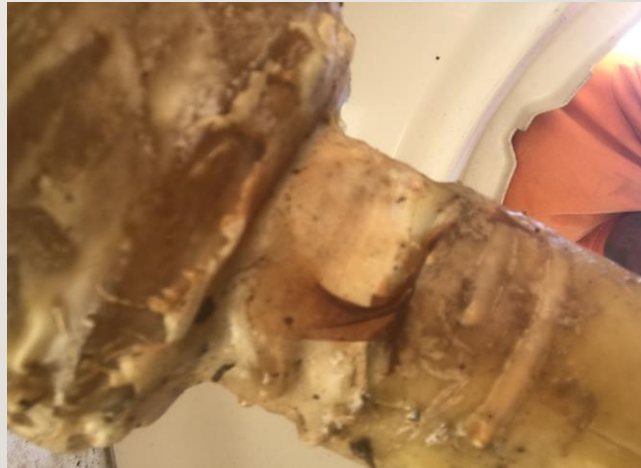
Same penetration fitting. Factory plug resin covered.
