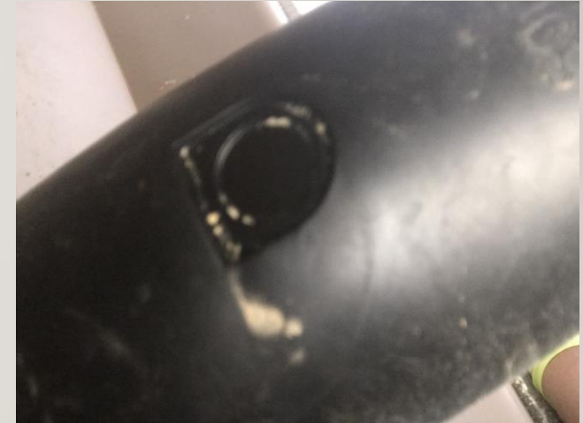
Designed to be at end of pipe run. Did they test IT properly?
