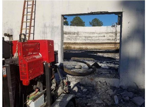
Completed access way in ET-10
