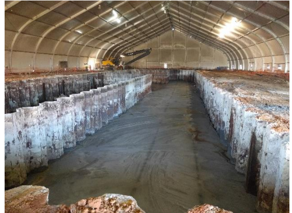
Barrier installation inside IB
