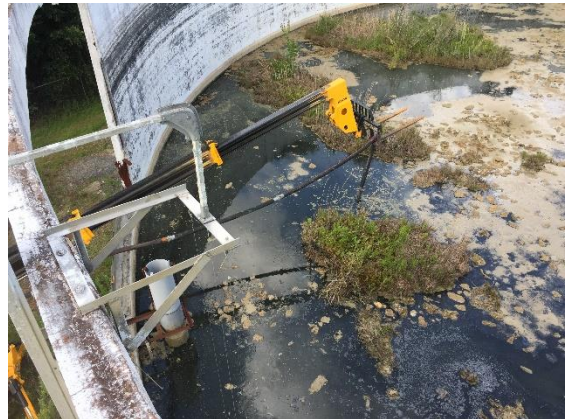
Pumping material from inside ET-10
