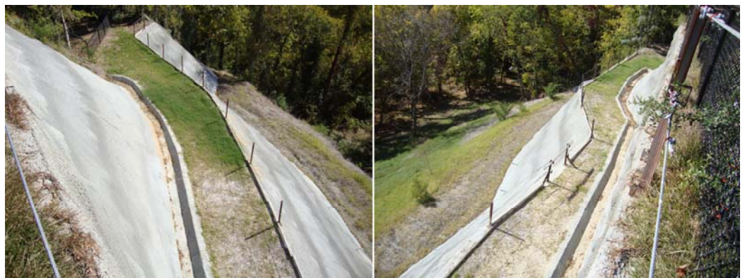
Figure 4. Views from the top of the retaining walls adjacent to the Mint Spring Bayou waterfall at the Vicksburg National Cemetery. Pictures were taken on October 29, 2011.
