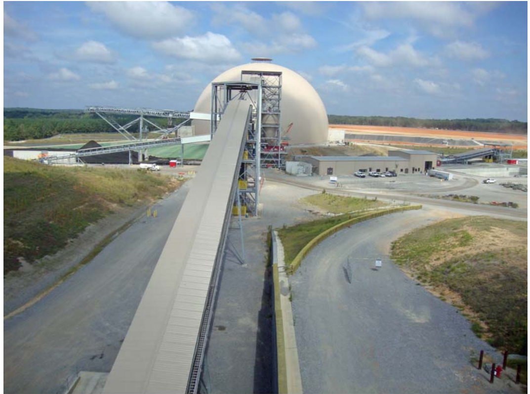
Figure 7. Covered conveyer belt and storage dome for lignite at the Kemper County mine and power plant. Picture was taken on September 30, 2014.
