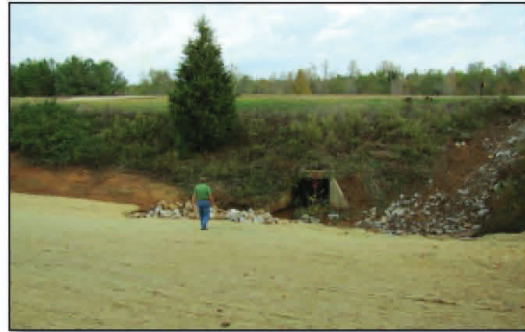
Figure 3. Critical area planting along Caney Creek was necessary to establish permanent vegetation on sites that had high erosion rates.
