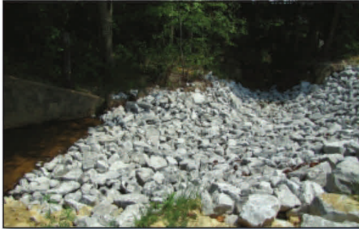
Figure 2. Grade stabilization structures in Caney Creek were used to prevent erosion and enhance the environmental quality of the creek.
