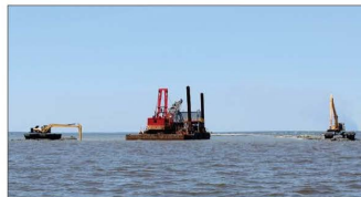
Construction of Round Island started in March of 2016.
