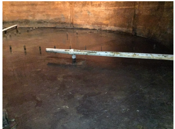
ET-18 after all material removed
