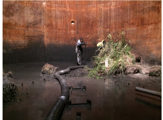
Removal of residual solids from ET-18
